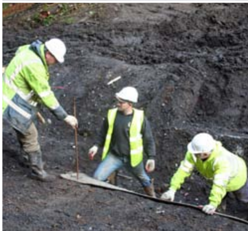
Pegging upper CC layer at 2m intervals
