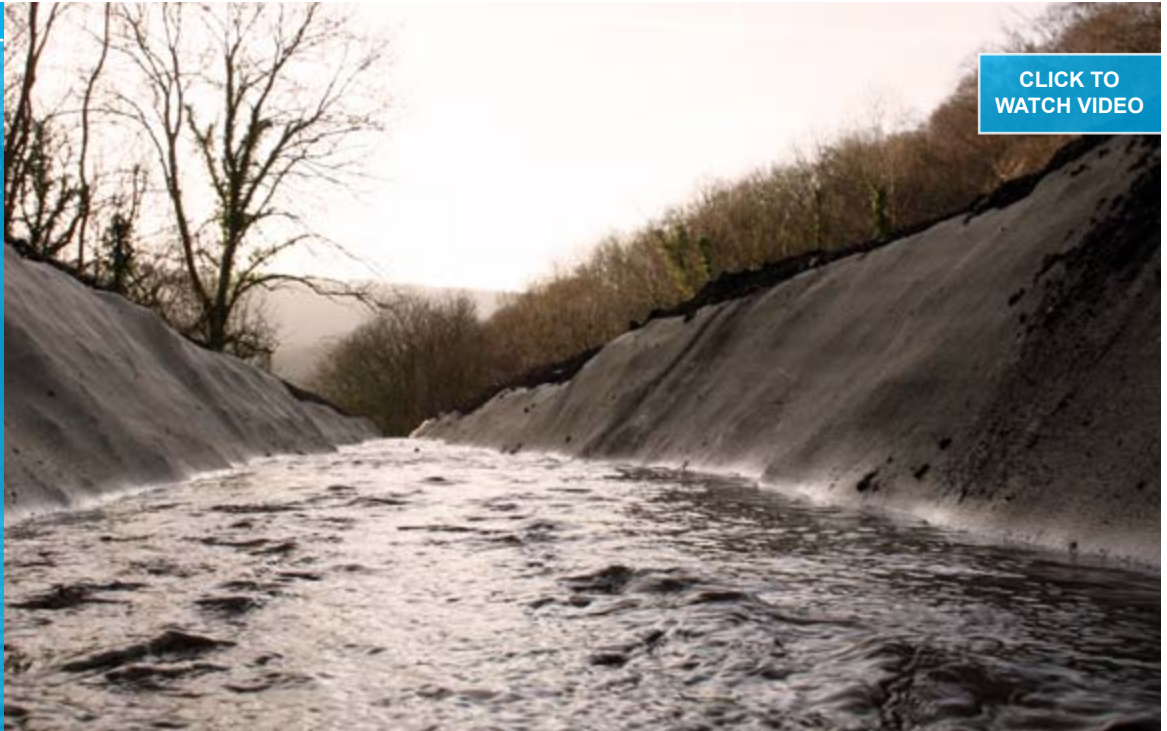
Completed two CC layer lined ditch channel with water flow
