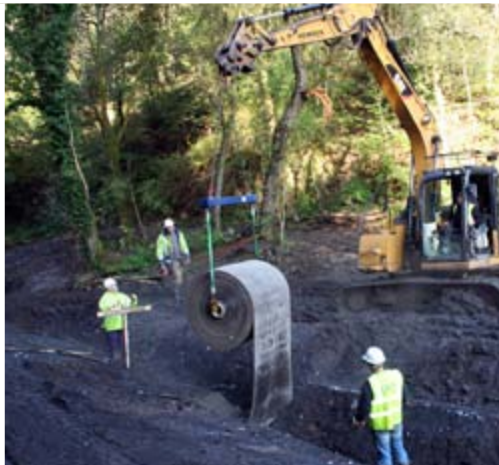
Dispensing CC bulk roll from spreader beam
