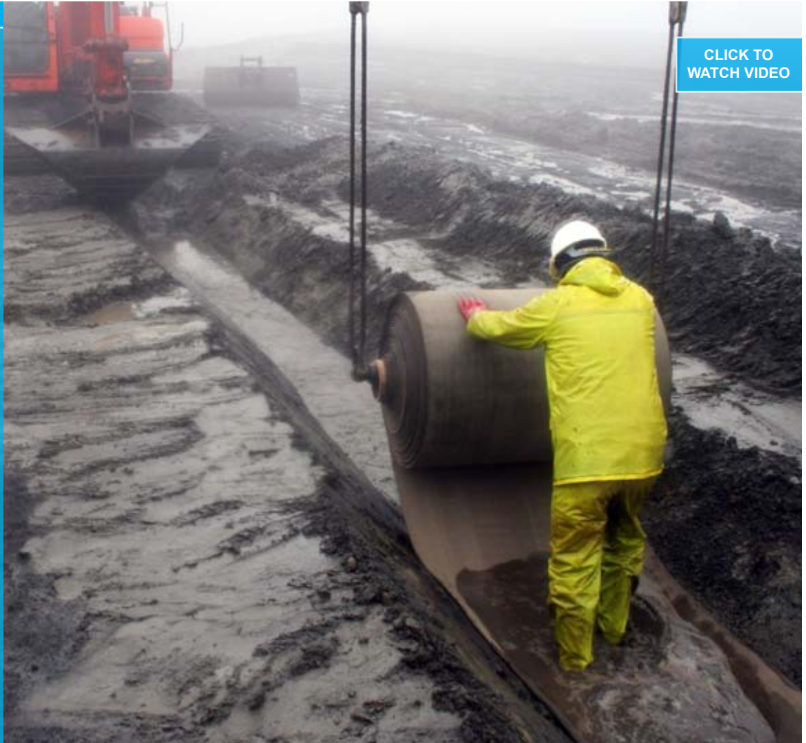
Installation of single layer of CC13 along channel in wet conditions
