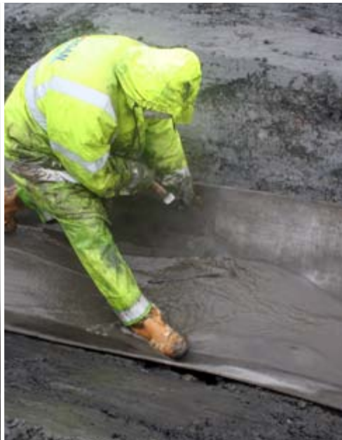
CC secured to substrate with pegs
