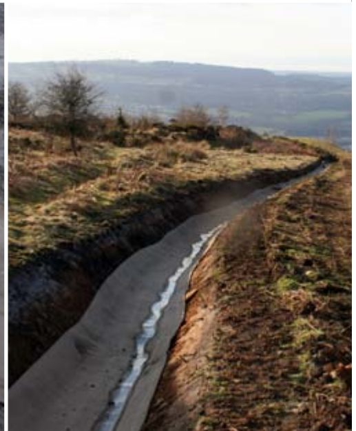
Completed CC lined channel
