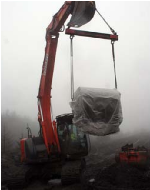
CC bulk roll transported to site
