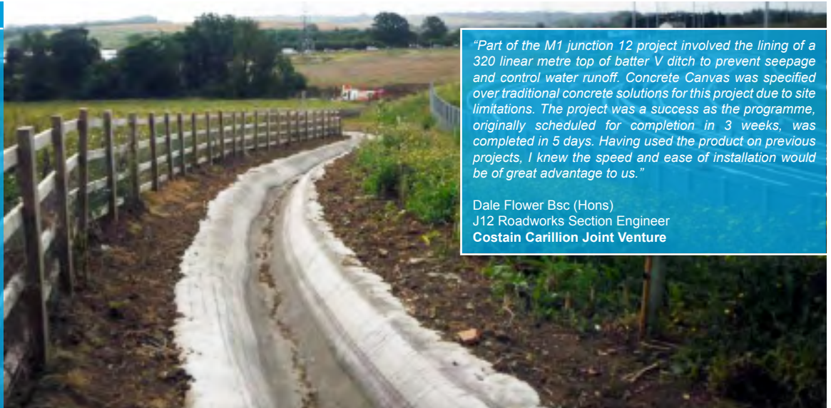
Completed lined ditch section
