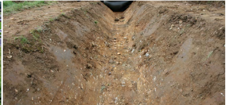
Graded ditch section with vegetation removed.
