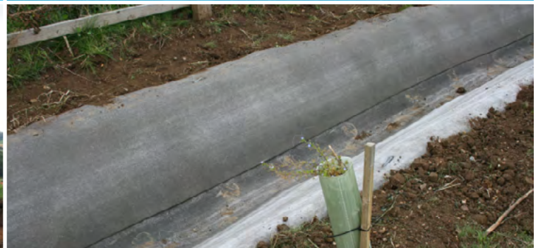
Completed CC lined ditch section secured with ground pegs at 2m intervals.
