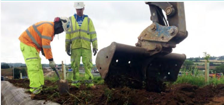
The edges of the CC were anchor trenched and backfilled after hydration.
