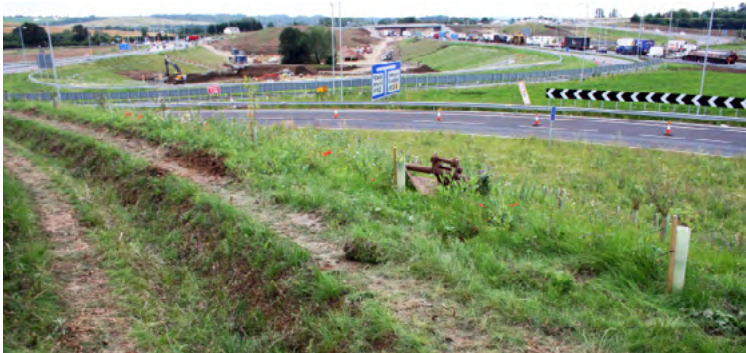
Batter prior to ditch excavation.
