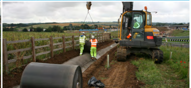
Lining the left side crest of the ditch
