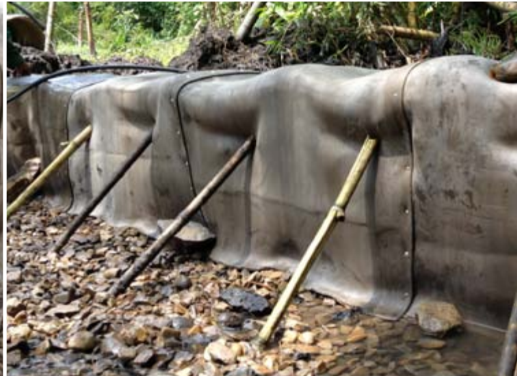
Wooden beams were used to close voids immediately after hydration
