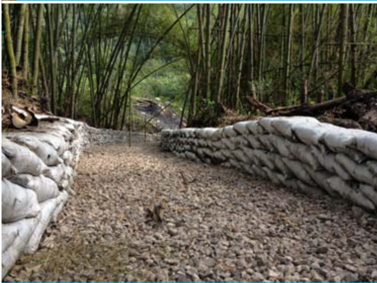
Ditch profile prior to lining with CC
