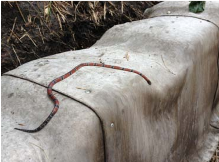
Adjacent CC layers were overlapped and screwed together
