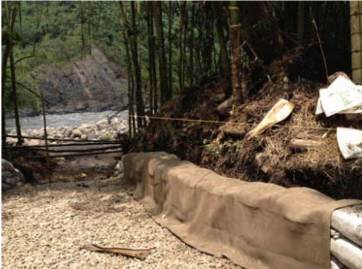
CC pre-cut sections of 1.5m positioned over sandbag wall prior to fixing
