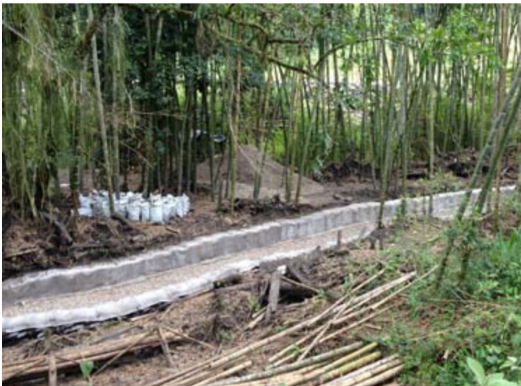
CC was applied to both sides of the 80 linear metre long ditch
