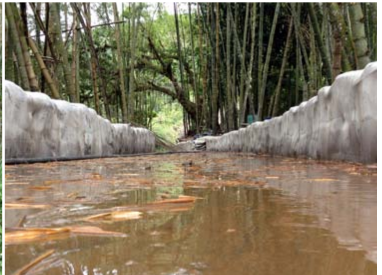
Completed CC lined ditch with redirected water flow
