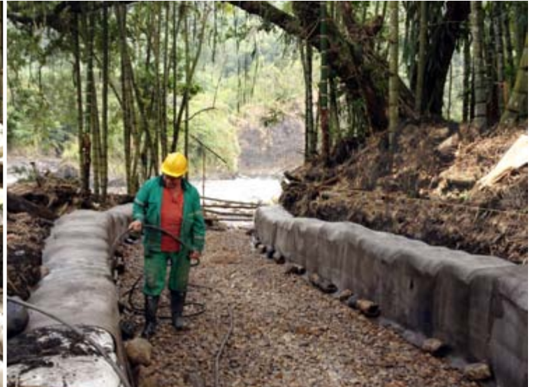
Hydration of the CC layers using local water source
