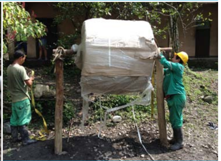
CC dispensed from a bulk roll on site before being cut to length
