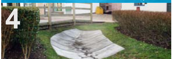
Completed CC lined swale
