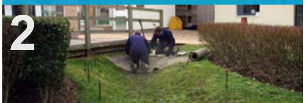
Laying and tailoring the CC to the swale profile
