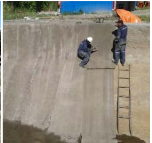
Fixing CC to the existing concrete substructure
