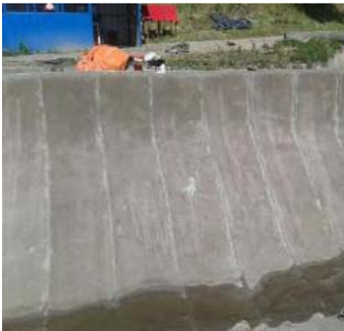
Lined concrete reservoir with sealed joints
