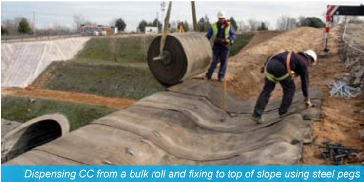
Dispensing CC from a bulk roll and fixing to top of slope using steel pegs
