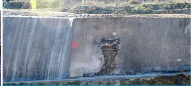
Damaged guniting section from previous remediation work
