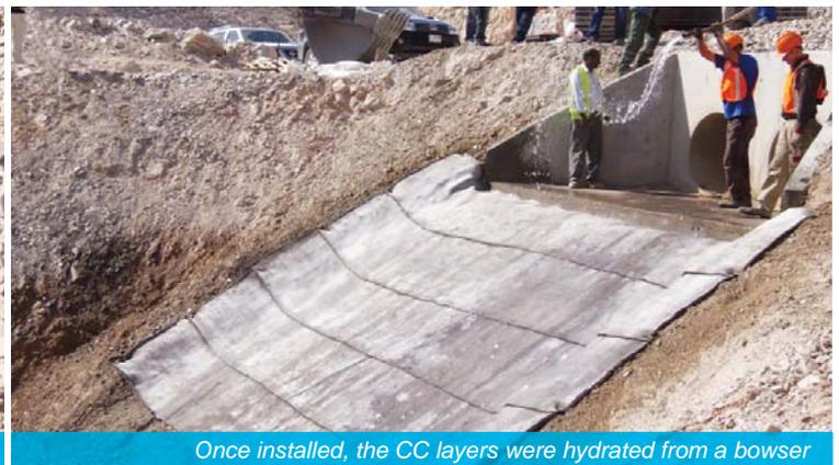
Once installed, the CC layers were hydrated from a bowser
