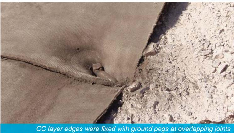
CC layer edges were fixed with ground pegs at overlapping joints
