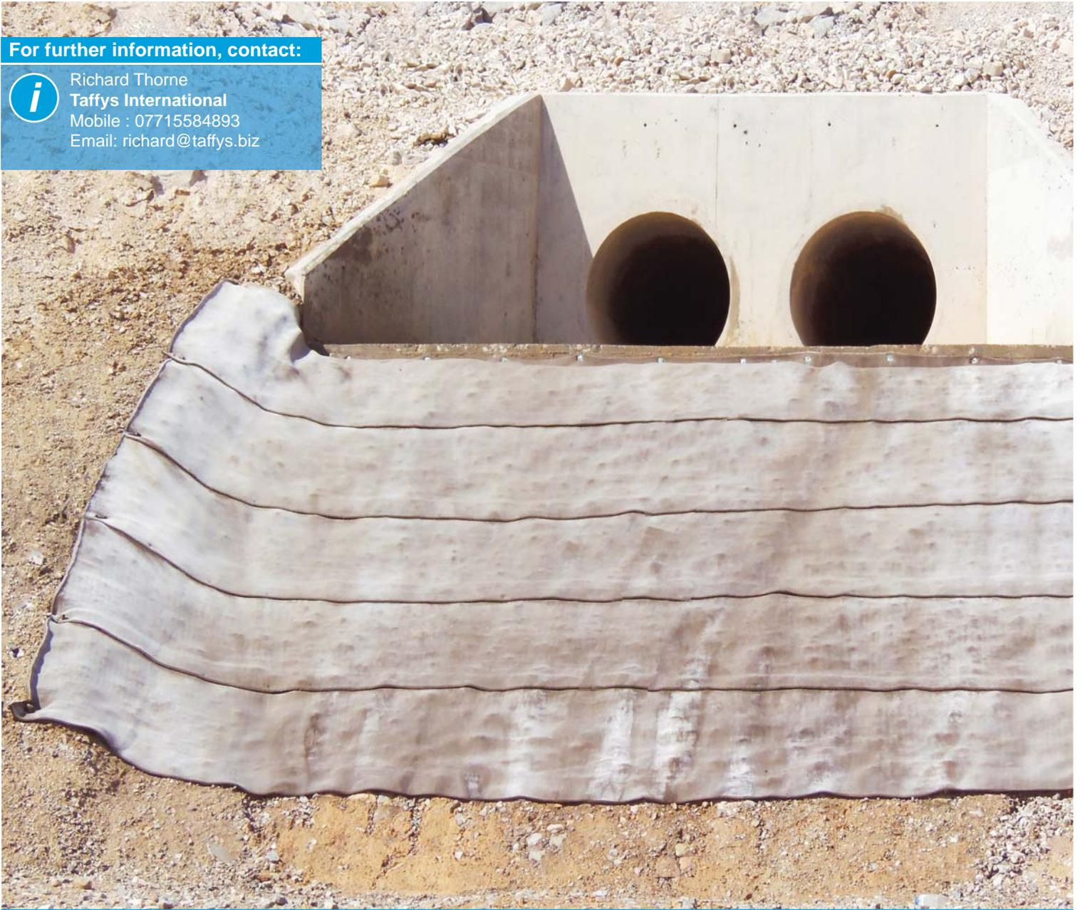
Completed CC slope protection installed in under 1 hour
