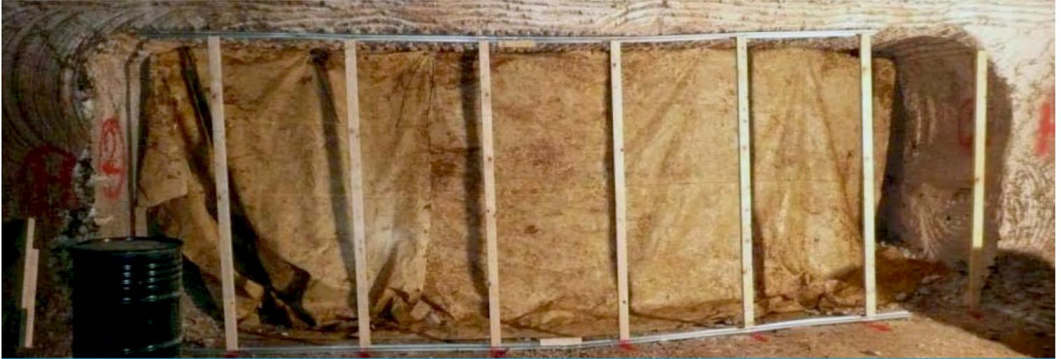
Frame created using British Gypsum branded aluminium stud wall system
