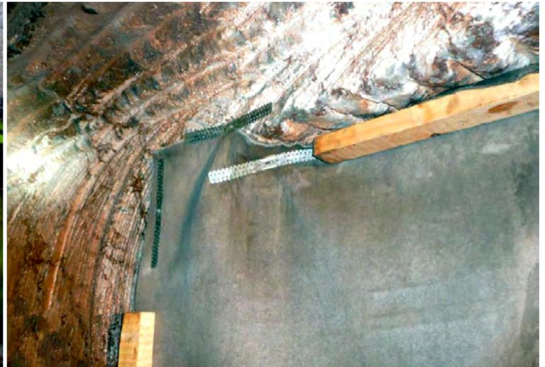
Battens, 200mm steel and screws used to provide strong fixing to rock
