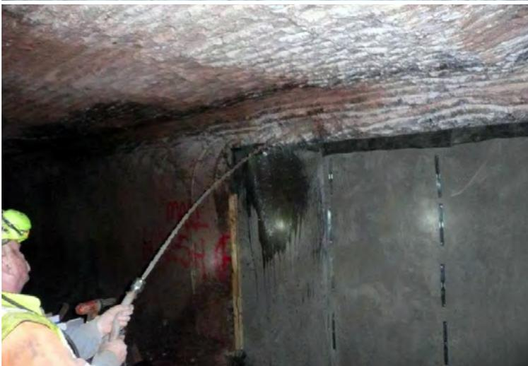
CC hydrated using on-site equipment
