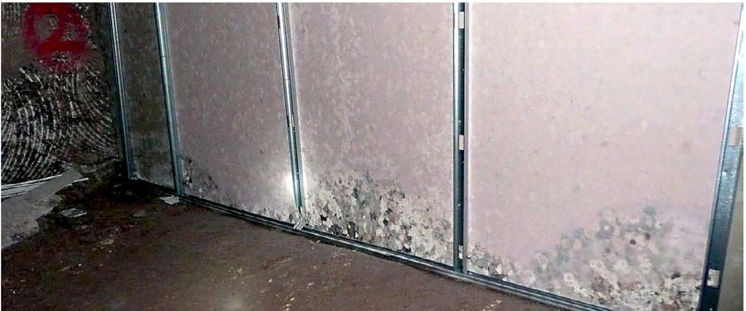
Vent walls had also been constructed out of the gypsum board the mine produced, but these were prone to rotting
