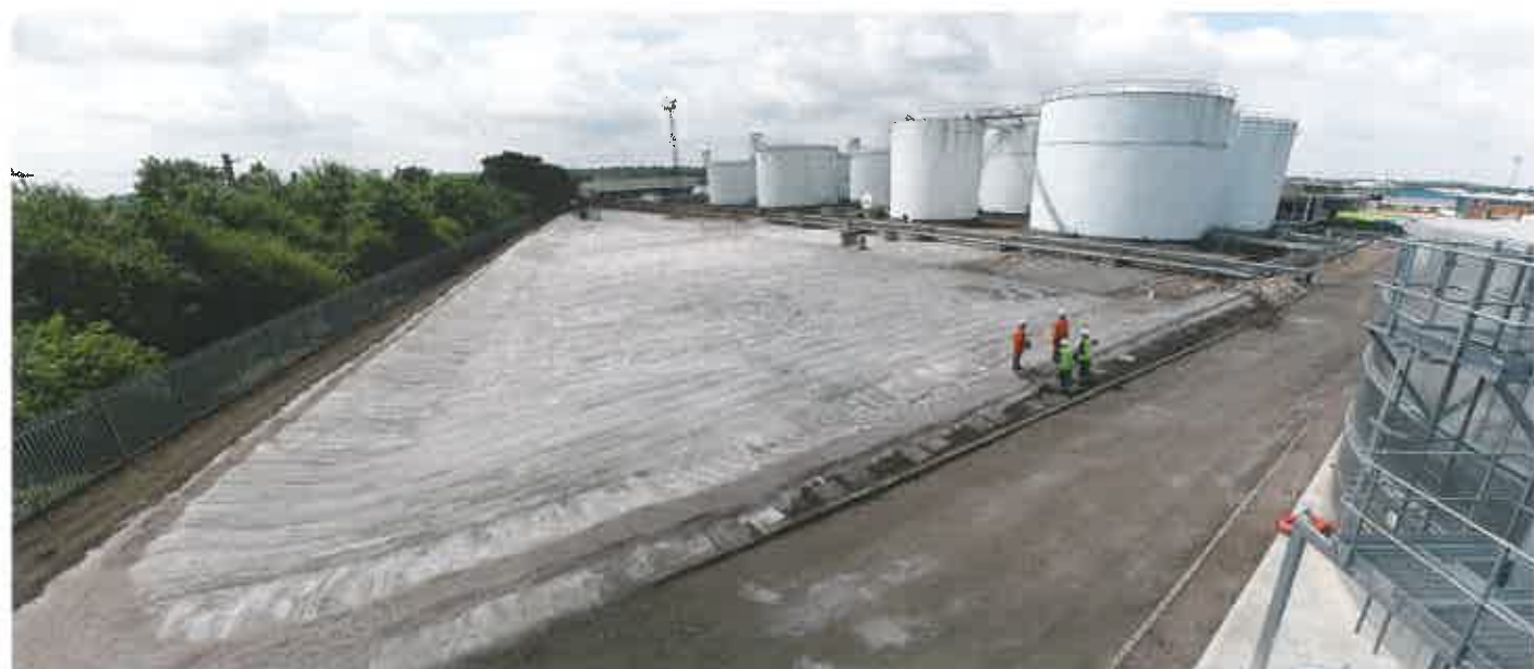
Completed installation of a lagoon lining
