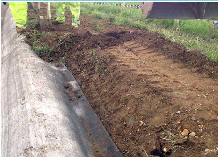
CC pinned in anchor trench which was then backfilled after hydration
