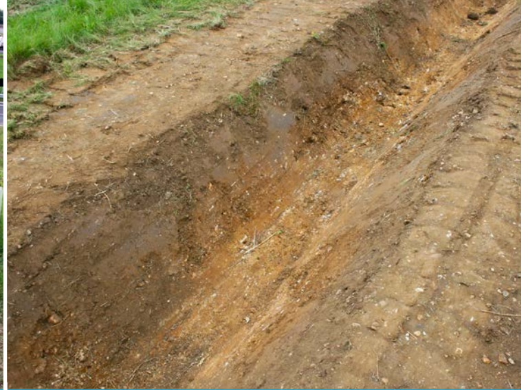
Graded ditch profile
