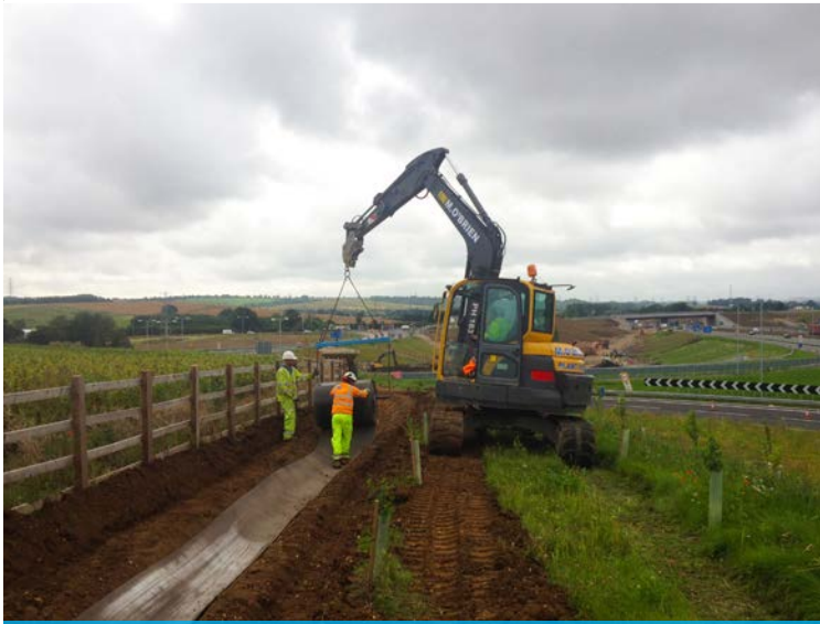
Deployment of CC via spreader beam
