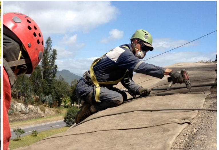
Adjacent layers of CC were overlapped by 100mm and screwed together
