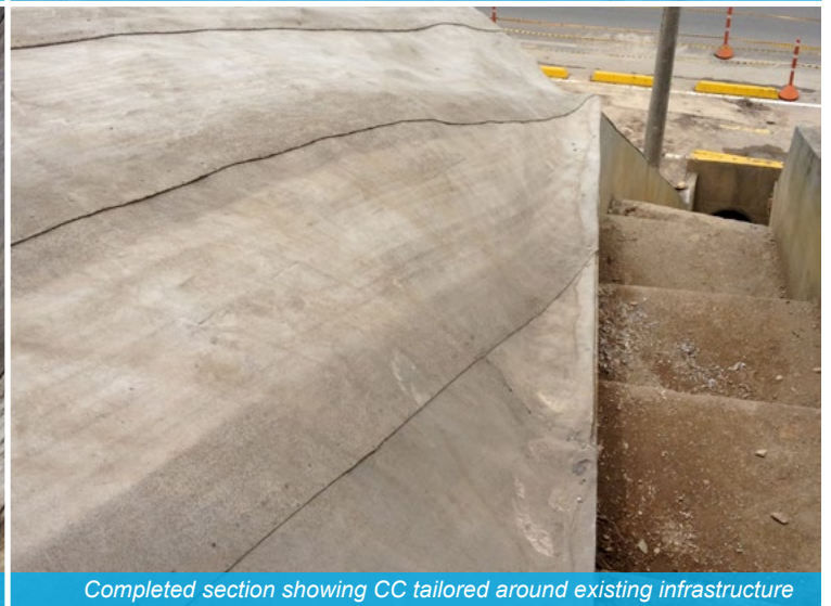
Adjacent layers of CC were overlapped by 100mm and screwed together
