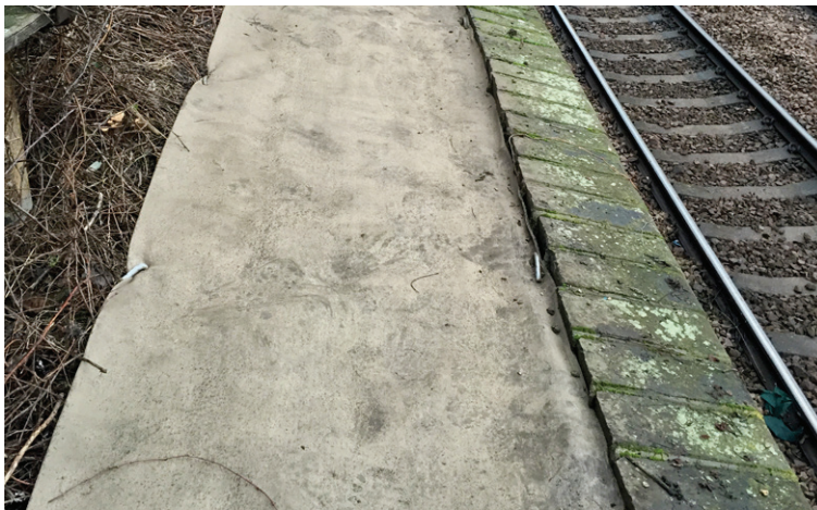
Fixing of the CC layers at 2m intervals using 250mm ground pegs
