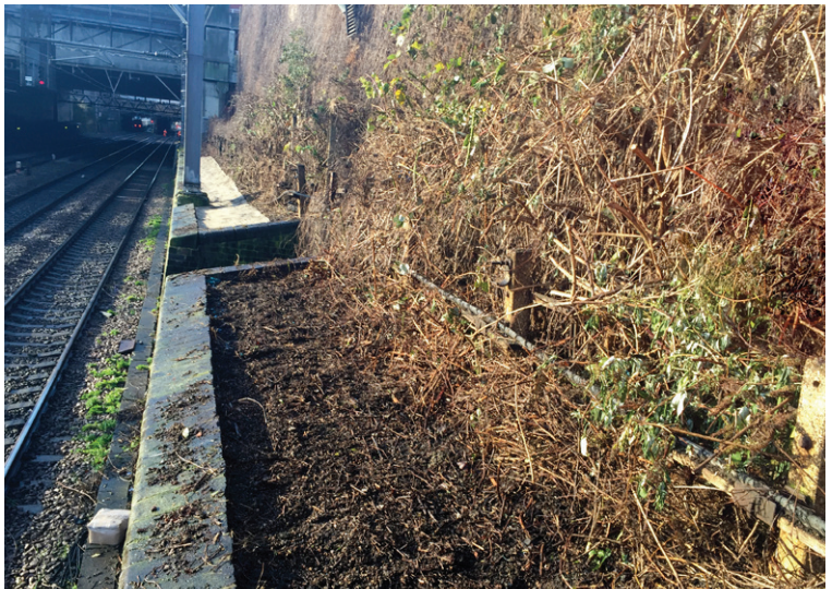
Parapet ledge cleared of vegetation and debris
