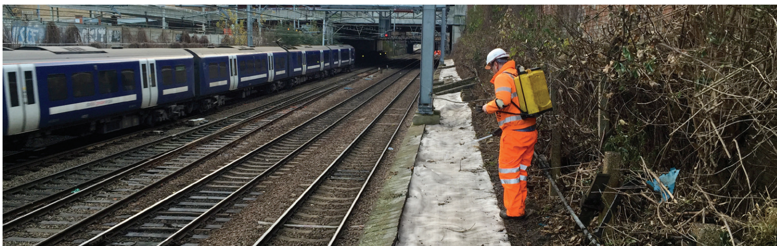
Backfilling anchor trench at toe of second section berm
