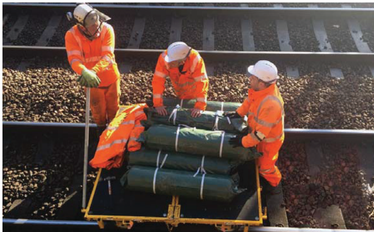
Delivery of CC batched rolls to site area via rail trolley
