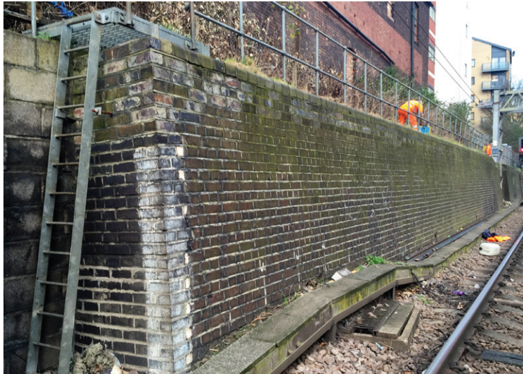
2.7m high signalling parapet to be weed suppressed
