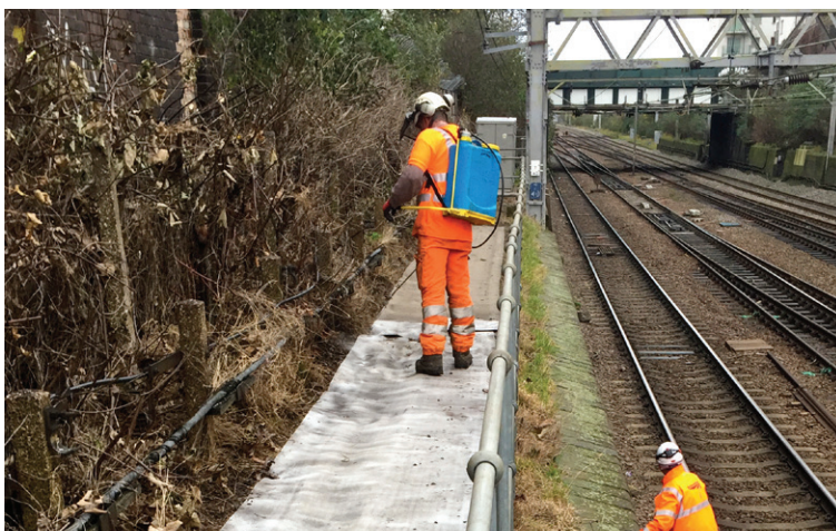
Hydration of the CC via 35l backpack sprayers
