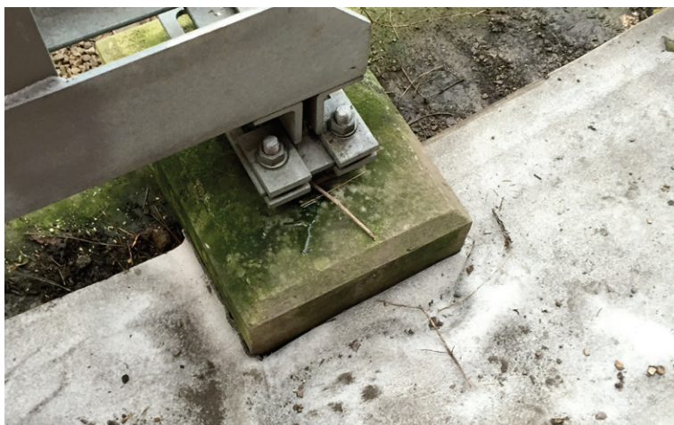
Cutting and detailing of CC to accommodate stanchions and upstands
