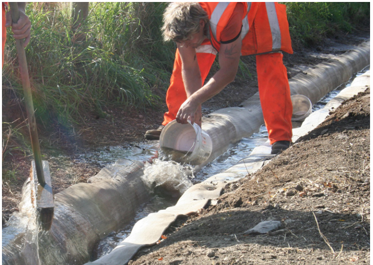
A bowser was used to fill the channel, which was further hydrated by hand
