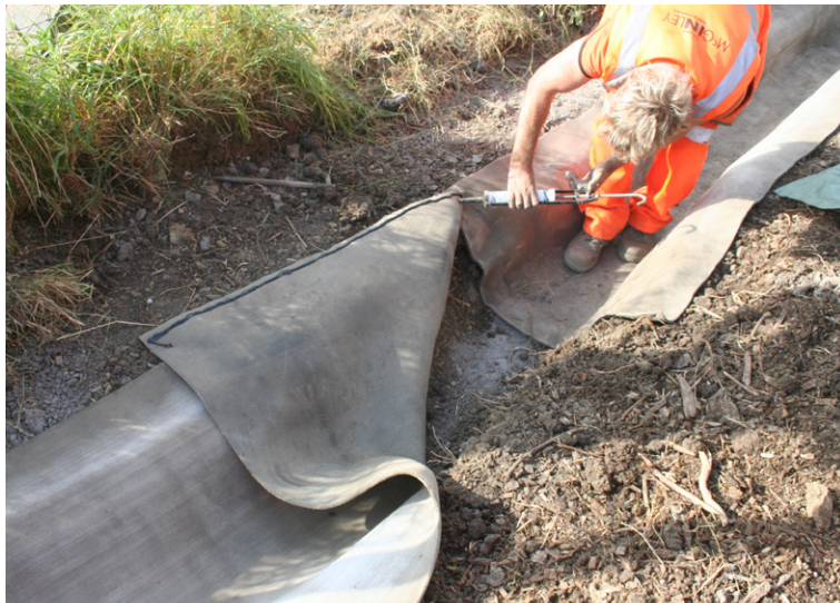
Sealant was used to fix the layers of CC together
