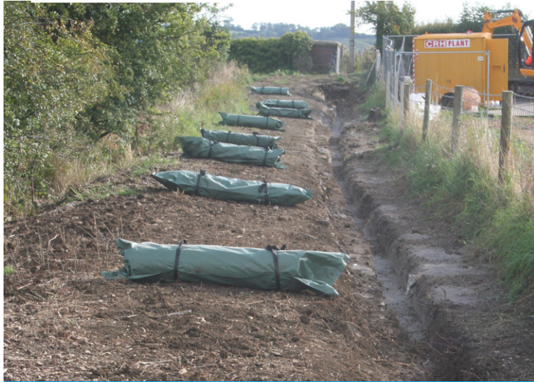
CC was delivered to site in batched rolls
