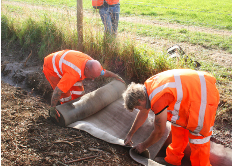
CC was laid longitudinally
