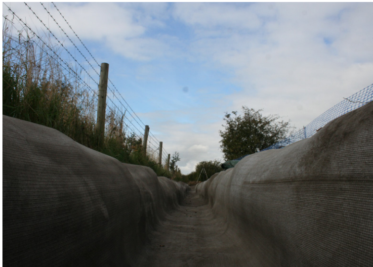
Completed installation, before hydration
