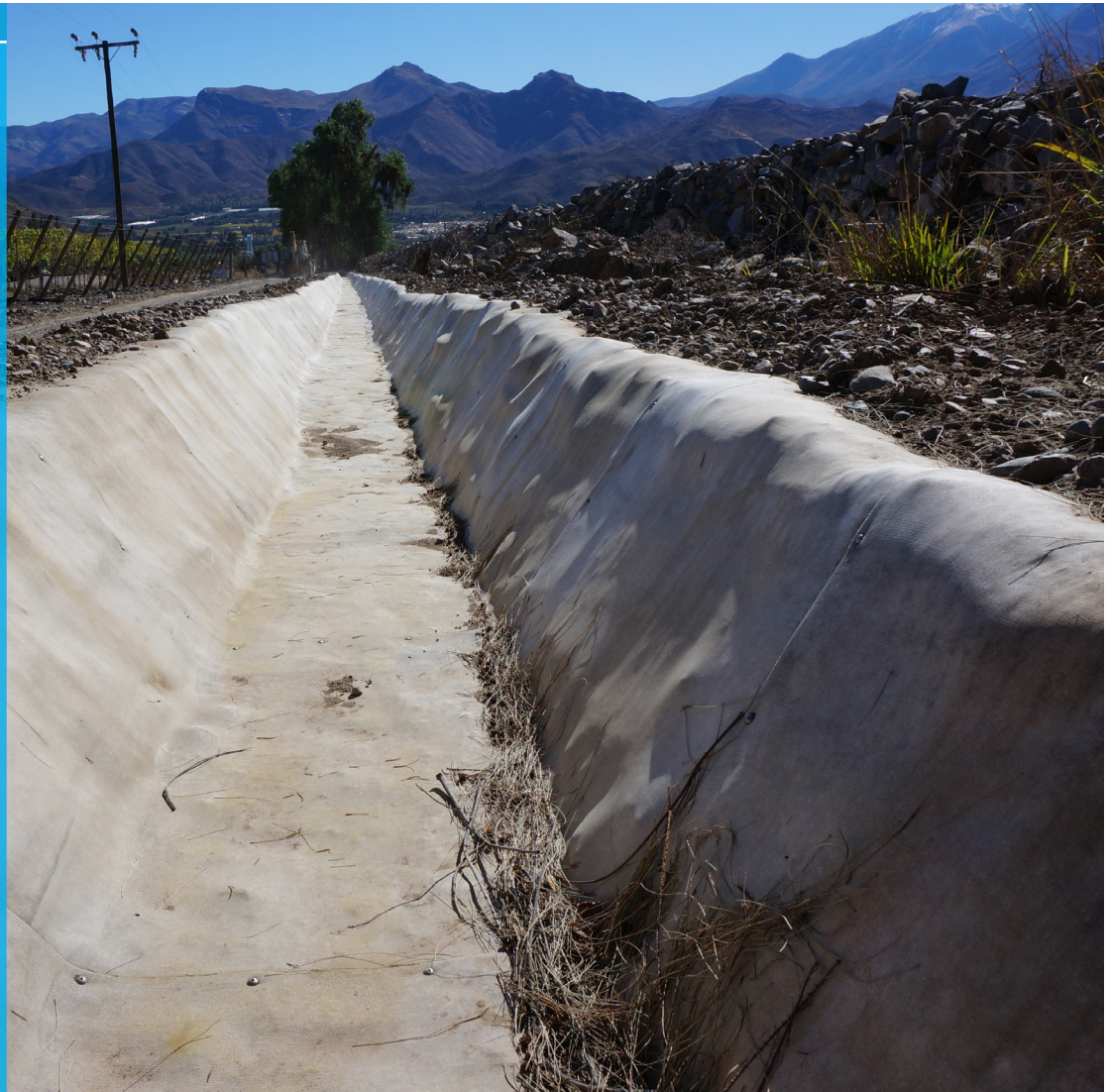
The completed installation after hydration, before water flow
