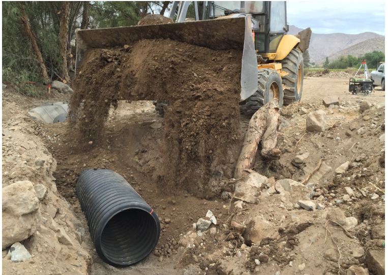
Pipes were installed underneath roads affected by the channel
