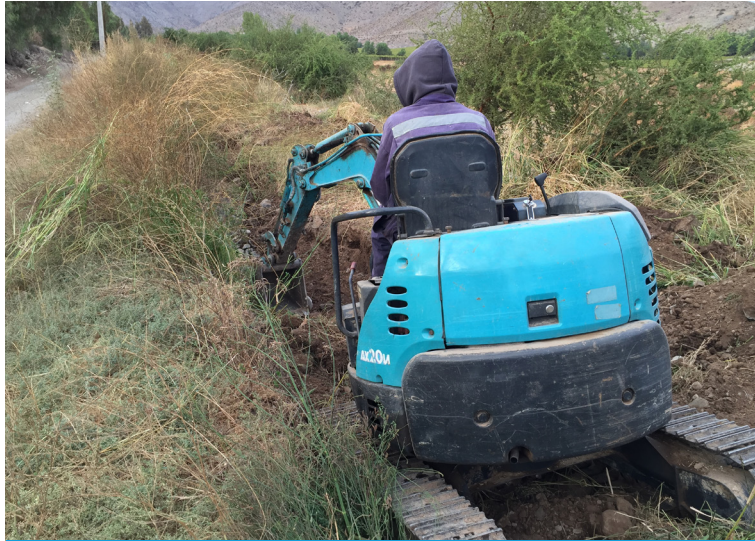
Vegetation was removed, excavated and levelled with a mini excavator
