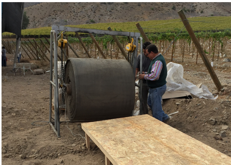
The CC was mounted onto a spreader beam and cut to the required length
