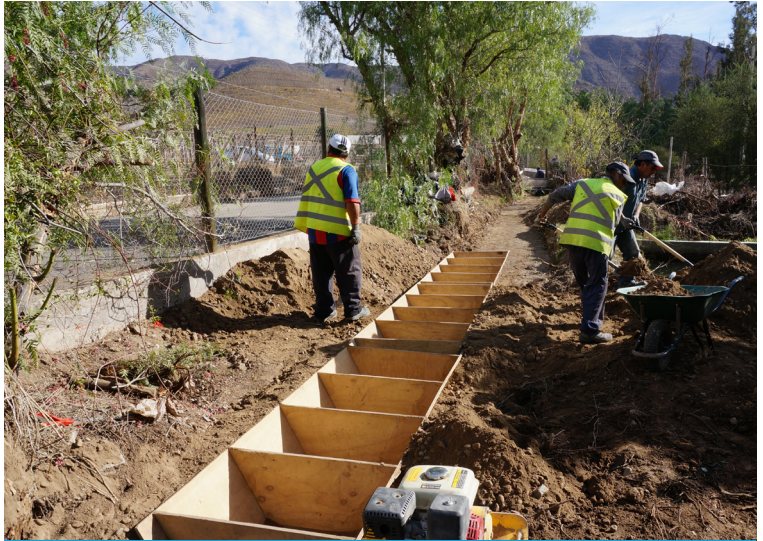
The profile of the channel was formed by the use of a wooden mold
