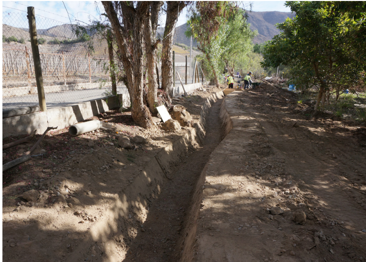
The complete graded channel profile
