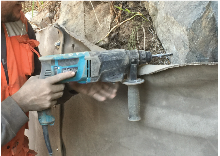
The CC was fixed to the natural rock surface with expansion bolts
