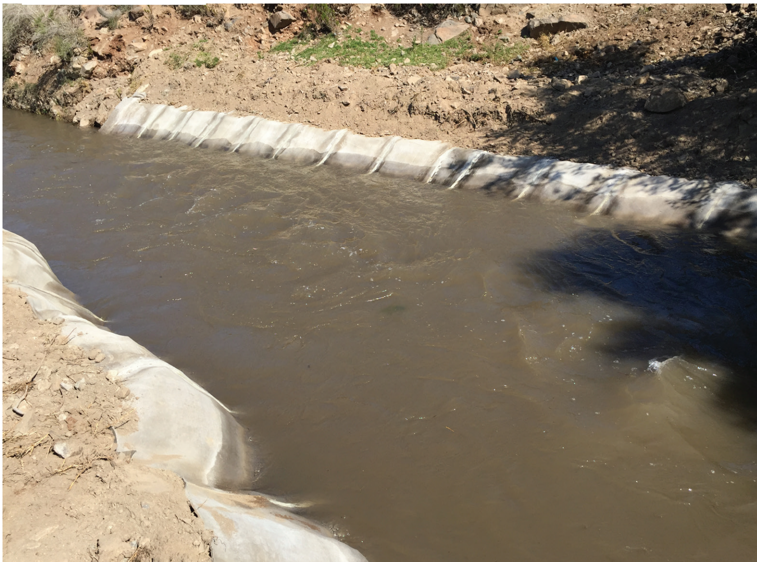
When in flow, there was a flow rate of 5.7m 3 per second within the channel
