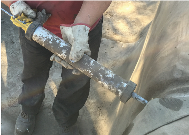
SIKAFLEX - 11 FC was used on each 100mm overlap
