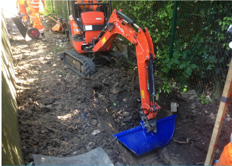
A Mini Excavator being used to grade the Channel profile
