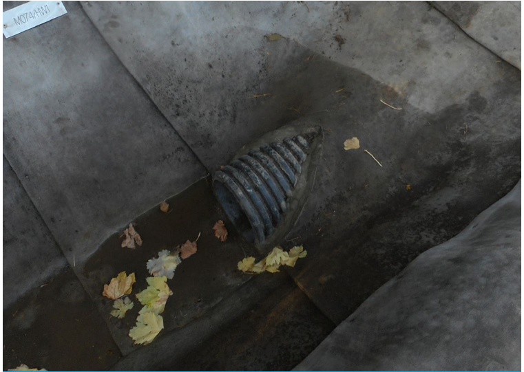
Any protrusions were grouted to provide a neat finish
