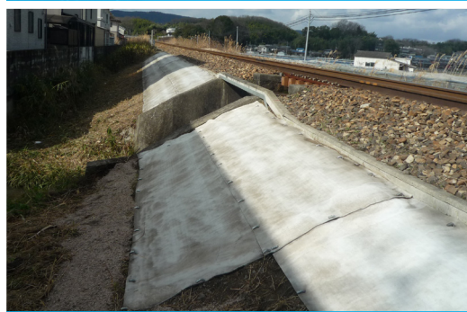
Layers of CC were overlapped by 100mm
