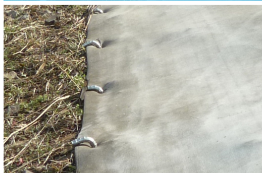
Ground pegs were used to secure the CC
