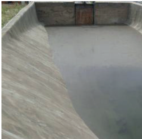
Refilling the basin to hydrate the CC
