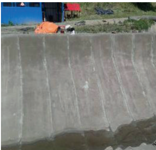
Lined concrete reservoir with sealed joints
