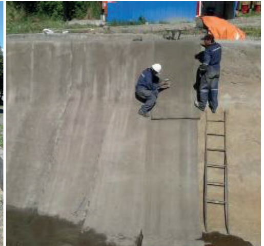
Fixing CC to the existing concrete substructure
