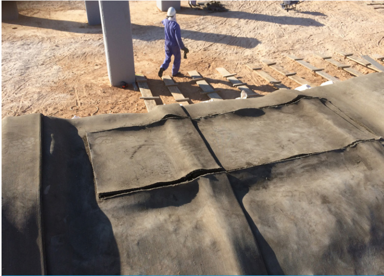
Cutting out the 100mm offset of plinth through laid up CC
