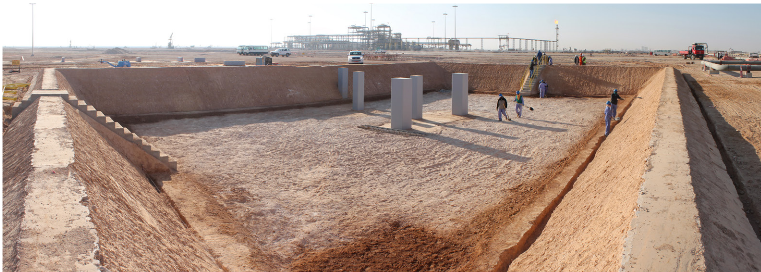
Excavated blow down pit prior to lining, with anchor trenches along inner and outer perimeters
