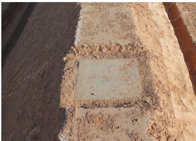
Concrete plinth for mounting pipework
