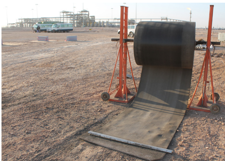
CC bulk roll on dispensing trolleys for cutting to batched lengths
