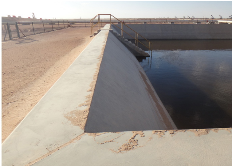
Conventional poured concrete blow down pit
