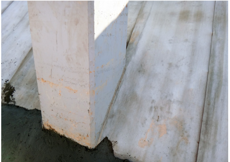
CC edges lapped, fixed and grouted to pillar face
