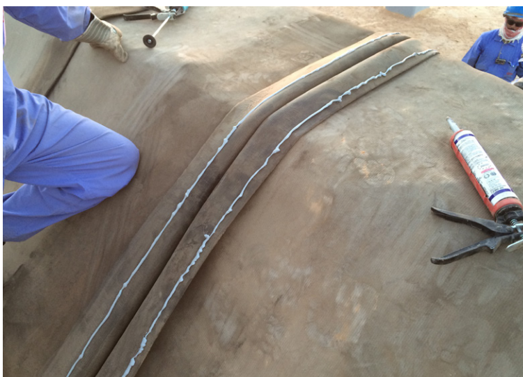
6mm continuous double beading on the PVC faces
