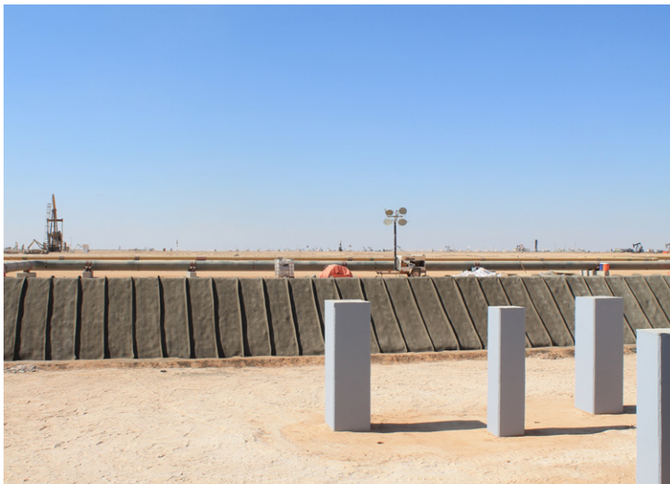
Thermal bonding on the berm face
