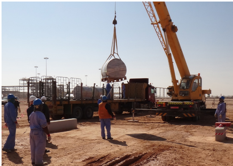
Unloading CC bulk rolls from the 40T flatbed delivery truck
