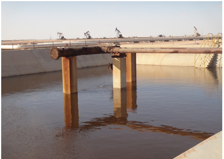
Steam condensing pipe manifold
