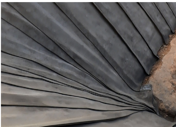
CT1 sealed corner detail prior to hydration and folding overlaps flush
