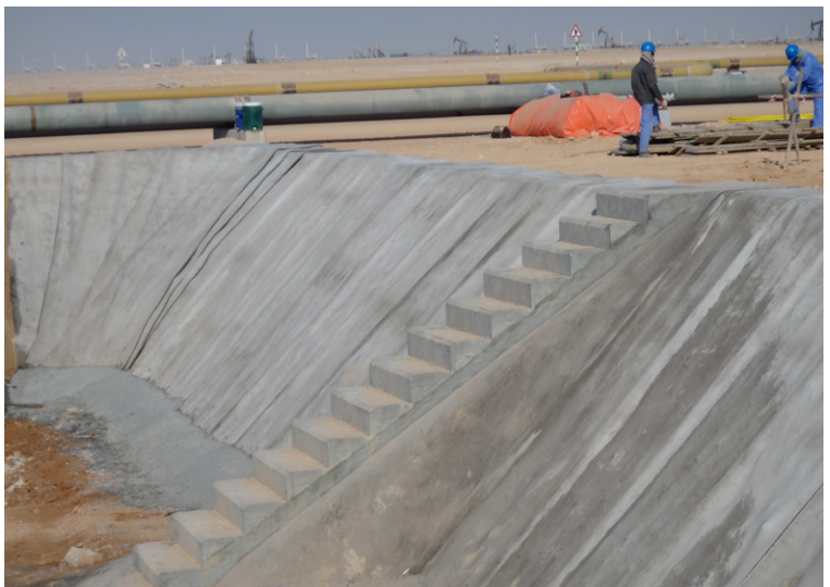
Completed stair section with grouted edges
