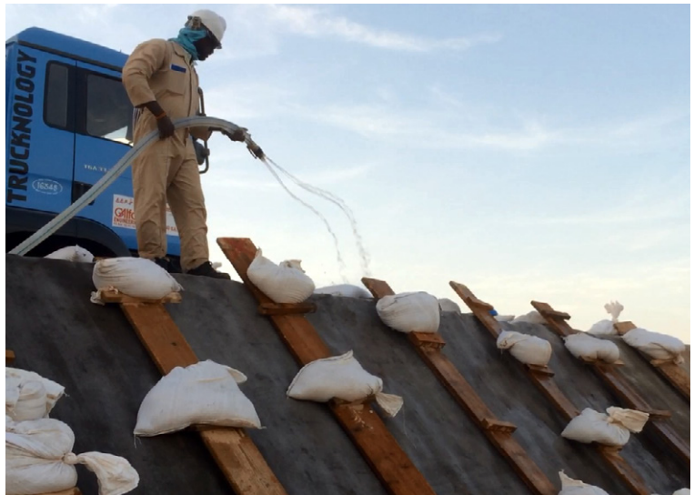
Sandbag weighted joints and hydration
