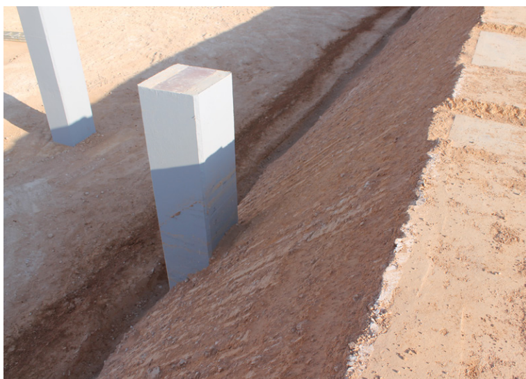
Concrete pillar inset into northern berm
