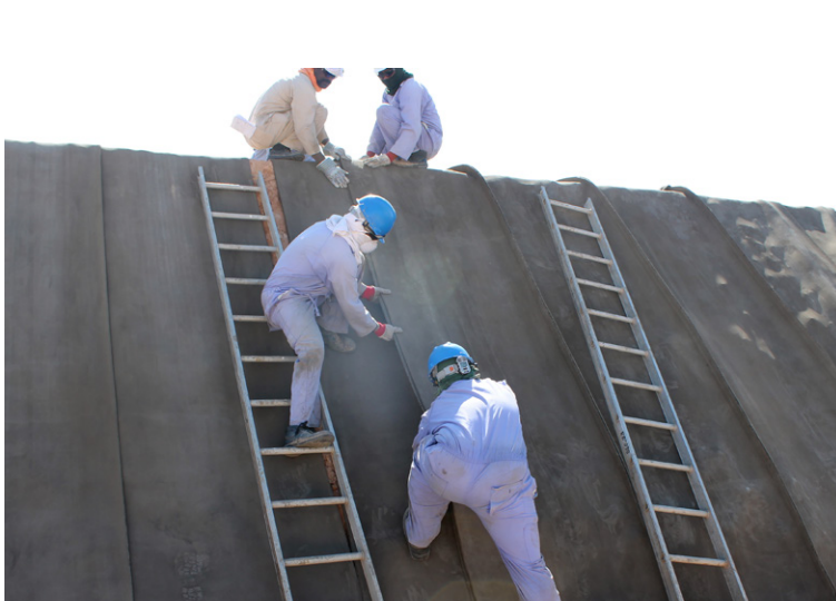
Positioning the man portable batched rolls of CC on the berms
