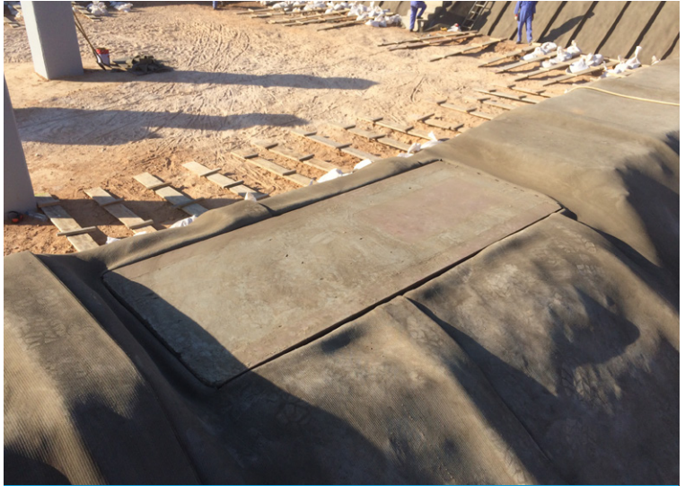
CC edges tucked into anchor trench to expose plinth
