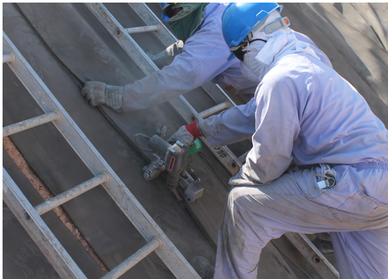
Thermal bonding on the berm face
