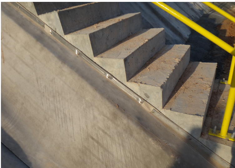
CC fixed to stair edge with steel strips
