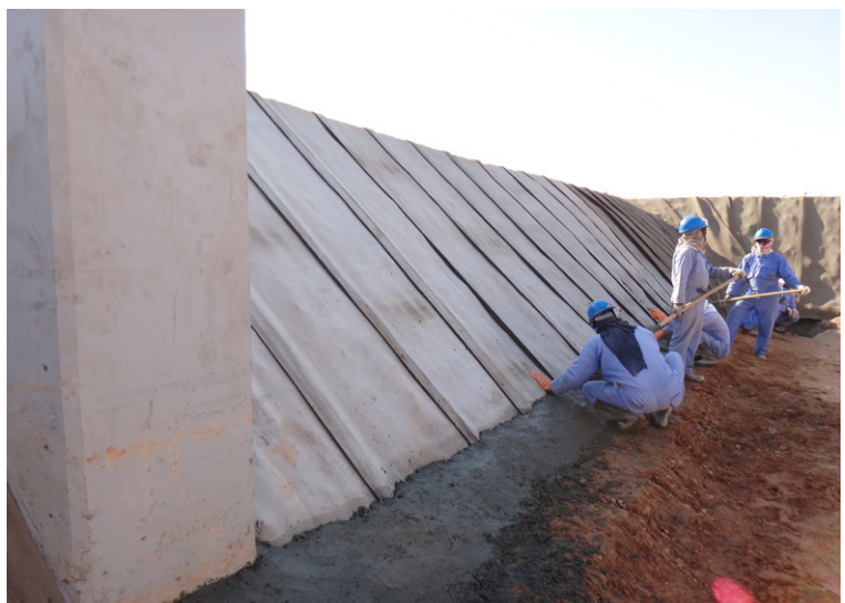
Applying concrete backfill
