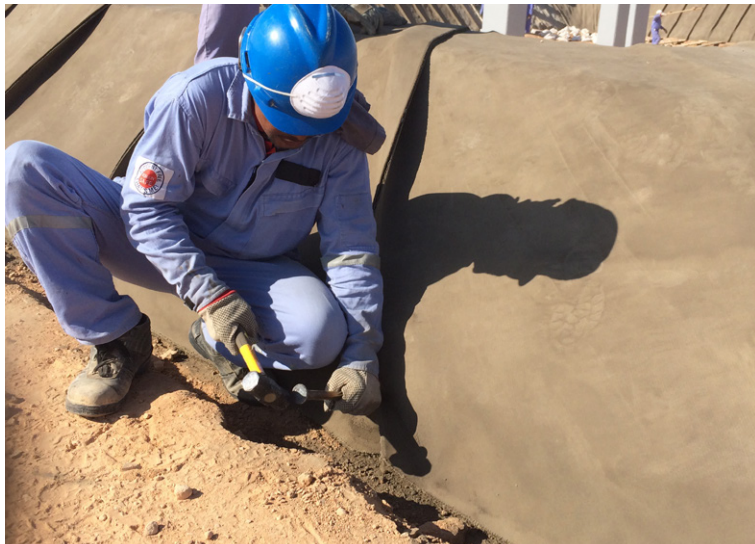
Fixing CC to the substrate
