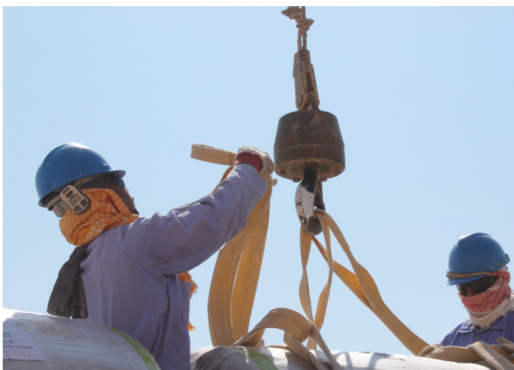
Unloading bulk rolls via lifting straps
