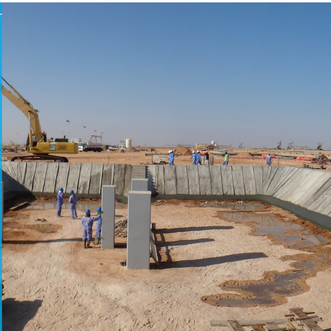
Completed, lined blow down pit
