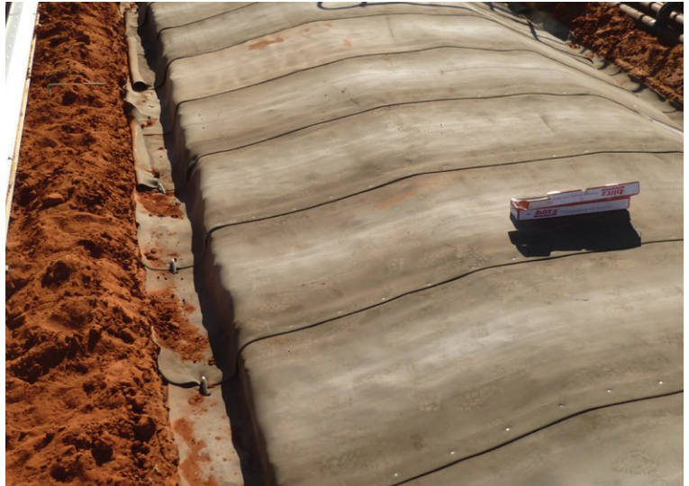
CC pegged in anchor trench and jointed with screws
