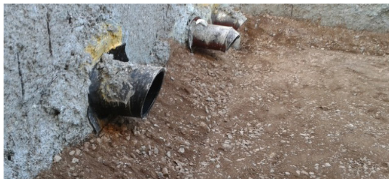
Recovering the tank ground level with graded earth
