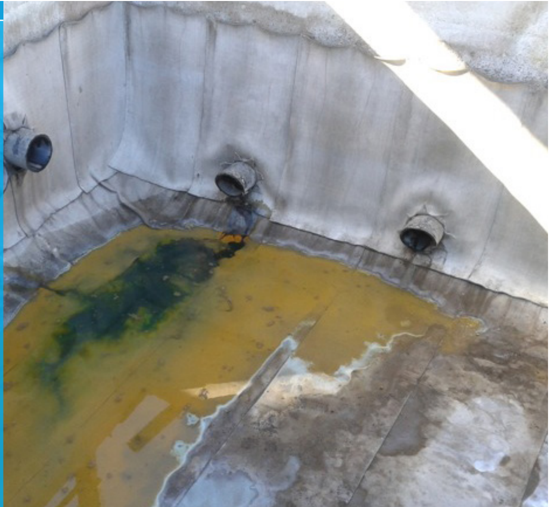
Completed lined acid tank 9 hours after hydration.
