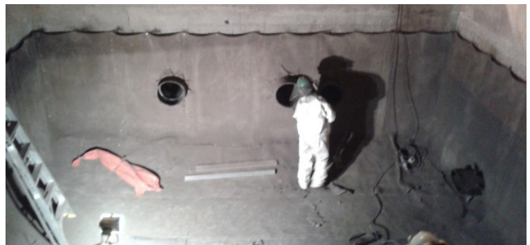
Completed installation (00:30 hrs)
