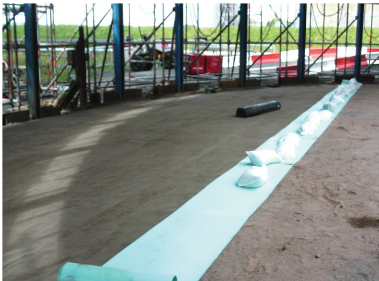
Leading edge of CCH5™ covered and held down with sandbags during hydration
