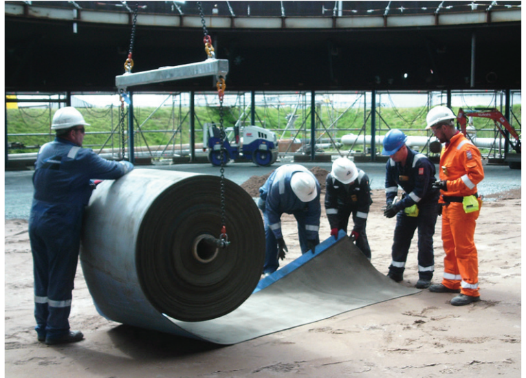
Deployment of the CC Hydro
