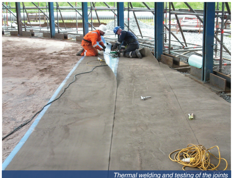
Deployment of the CC Hydro
