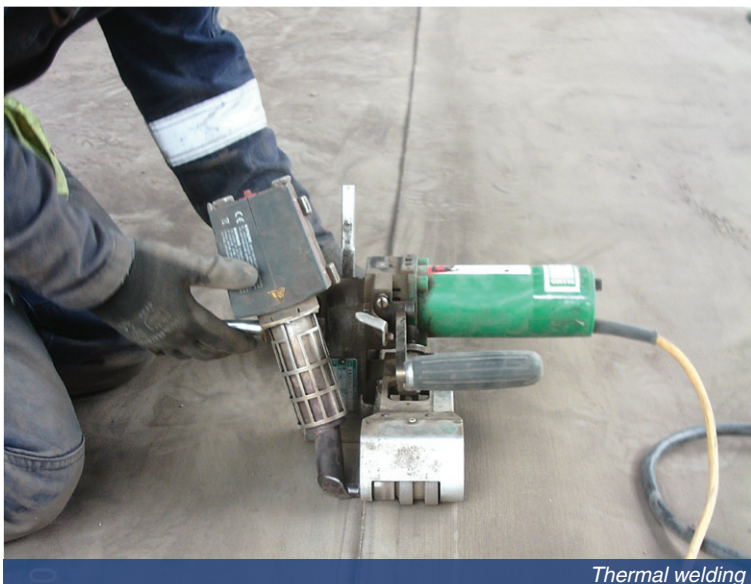
Testing the welding machine at the start of each day prior to installation
