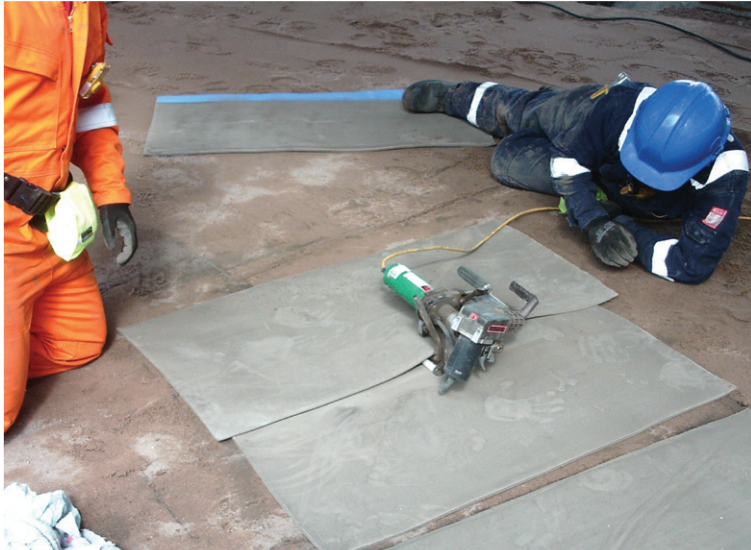
Testing the welding machine at the start of each day prior to installation
