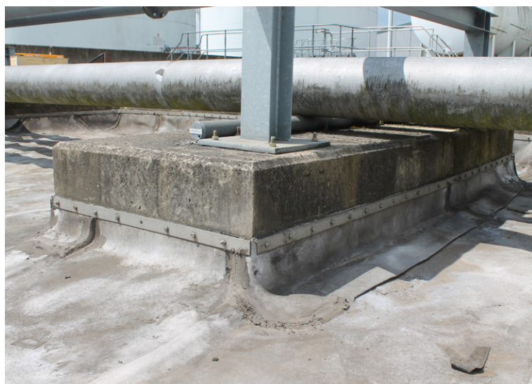
Grouted corner joints of concrete plinth
