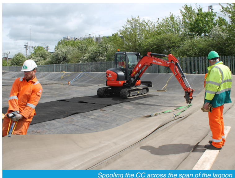
20T excavator manoeuvring a bulk roll to the lagoon centre
