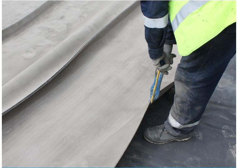
CC being laid directly onto the existing liner
