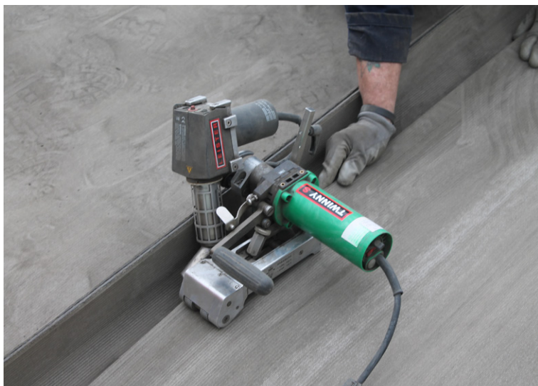
Thermal bonding of prayer joint
