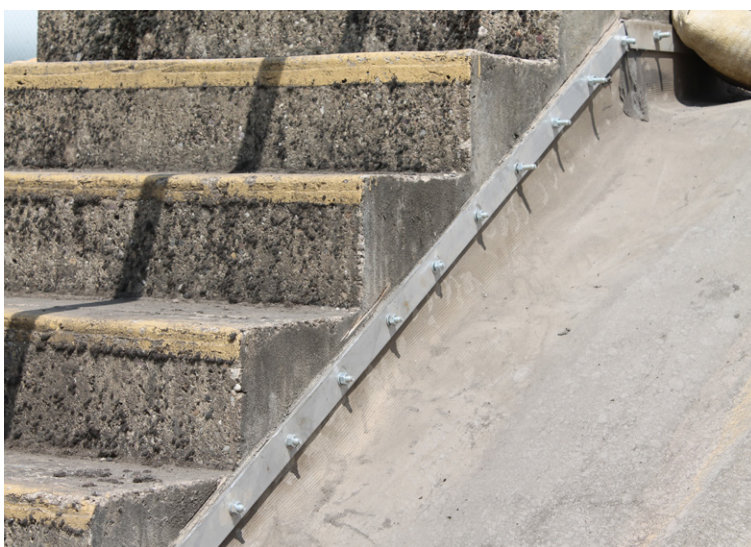
5mm plate with Fischer stud anchors at 100mm centres
