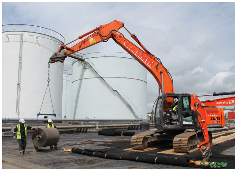
20T excavator manoeuvring a bulk roll to the lagoon centre
