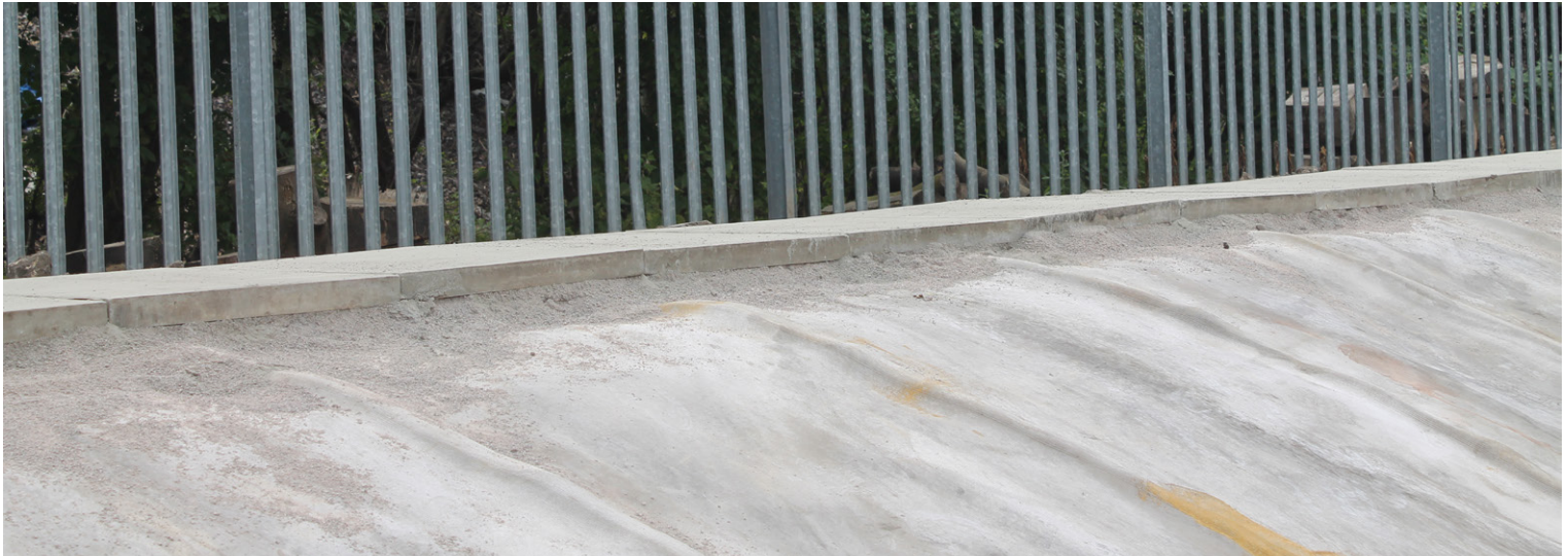
Edge finishing: replacement of flag stones and backfilling along palisade fence
