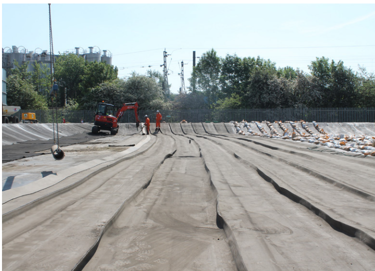
Welded joints prior to hydration and sandbagging
