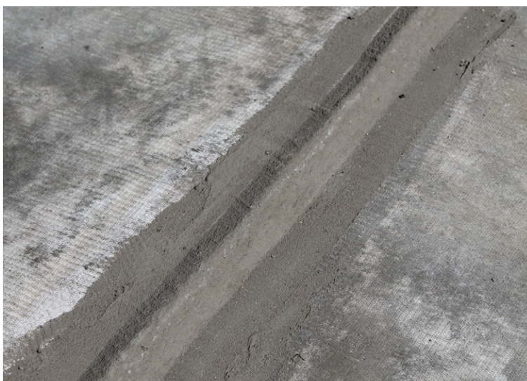
Grouted joints where welding not possible
