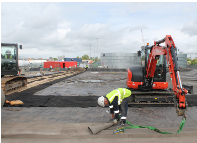
Attaching the leading edge of the CC to the 5T excavator
