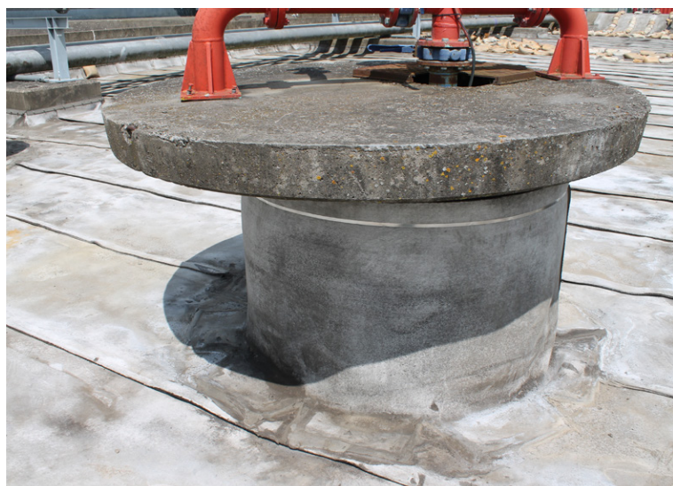
Hydrant up stand wrapped in CC collar secured at top with band
