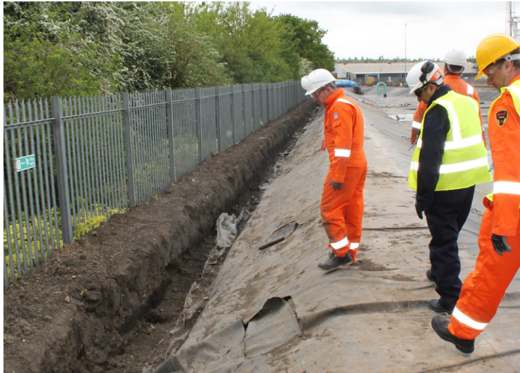
Excavated anchor trench
