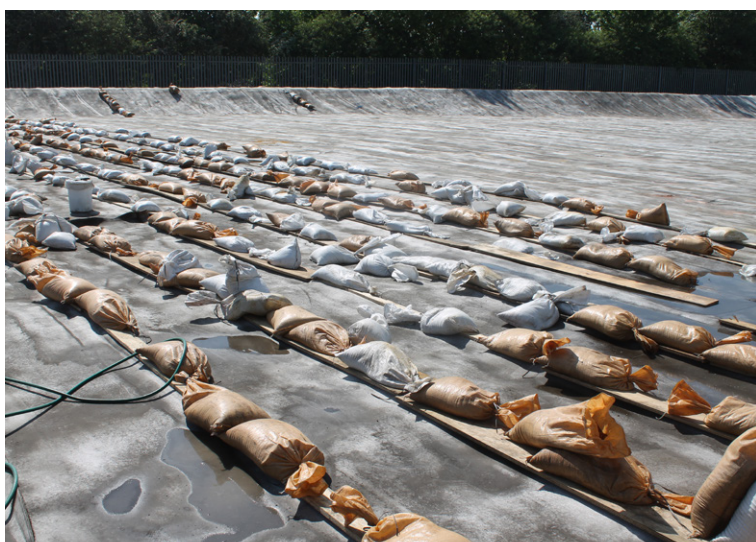
Joints weighted down after hydration
