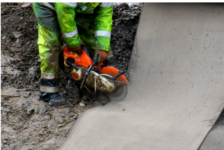
Cutting CC using a powered disc-cutter
