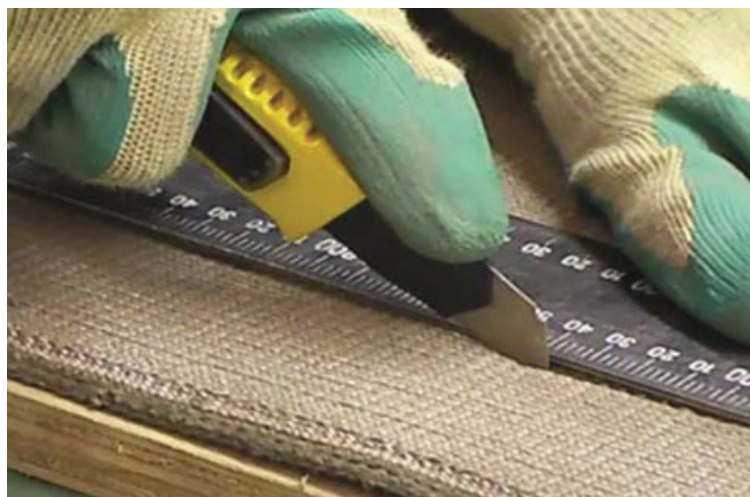
Cutting CC using a 'snap-off blade' utility knife
