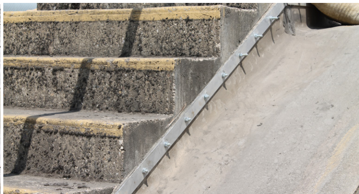
Pre-drilled galvanised steel bar fixing
