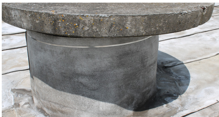
Clamping band fixing
