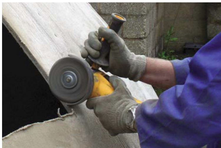
Cutting set CC using an angle grinder
