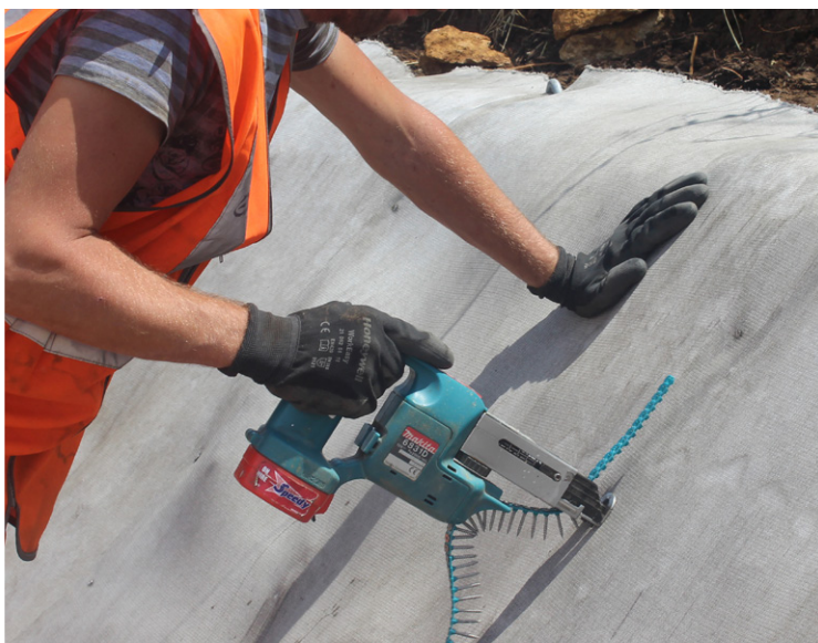
CC joint fixed using an autofed screwdriver
