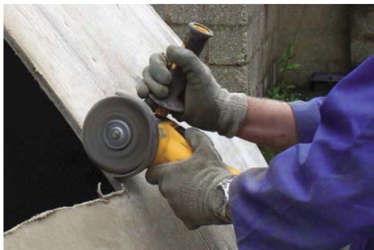
Cutting set CC using an angle grinder
