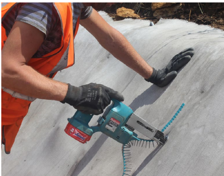
CC joint fixed using an autofed screwdriver
