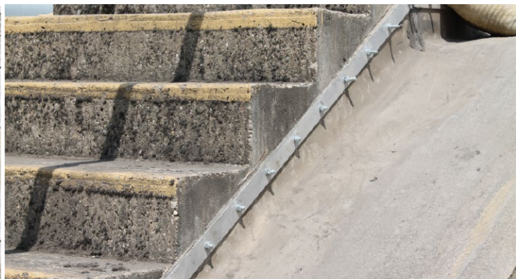
Pre-drilled galvanised steel bar fixing
