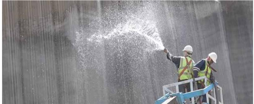
**SPRAY THE FIBRE SURFACE WITH WATER UNTIL IT FEELS WET TO TOUCH FOR SEVERAL MINUTES AFTER SPRAYING**
