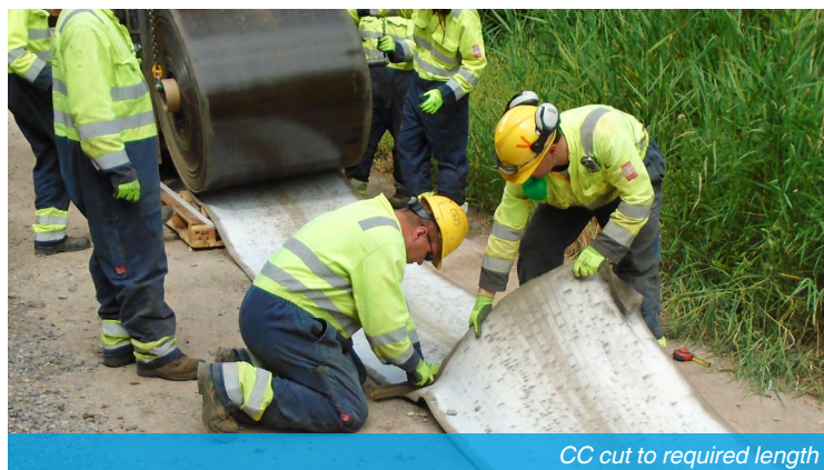
CC deployed using a low profile deployment frame
