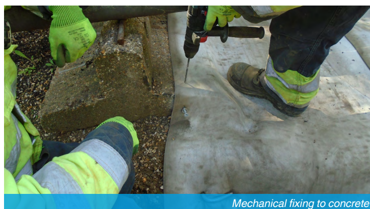
Mechanical fixing to concrete
