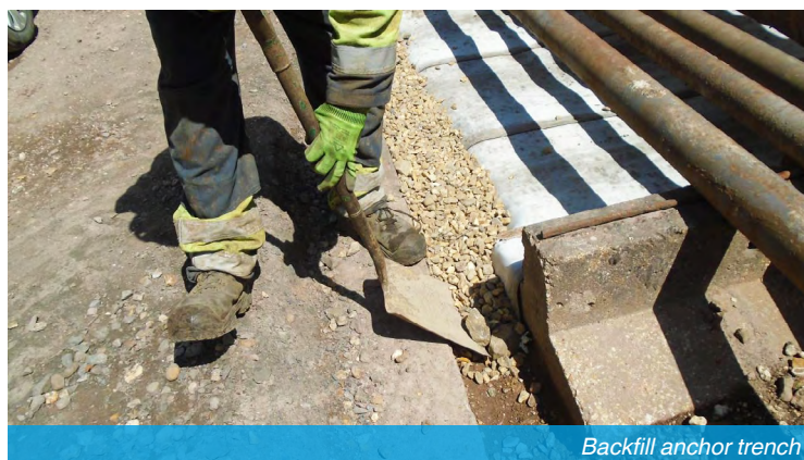
Anchor trenches should be a minimum of 100mm
