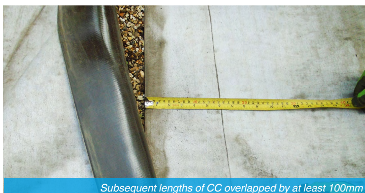
Subsequent lengths of CC overlapped by at least 100mm
