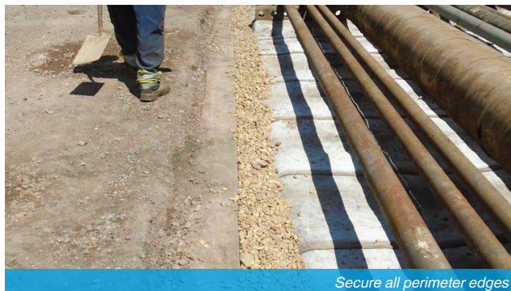
Backfill anchor trench
