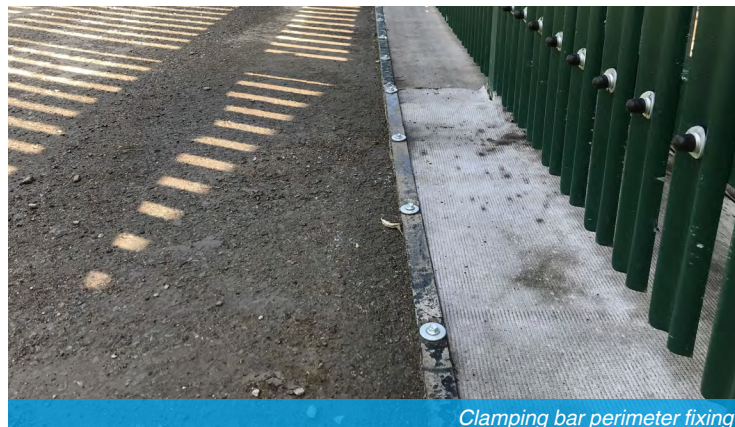
Clamping bar perimeter fixing
