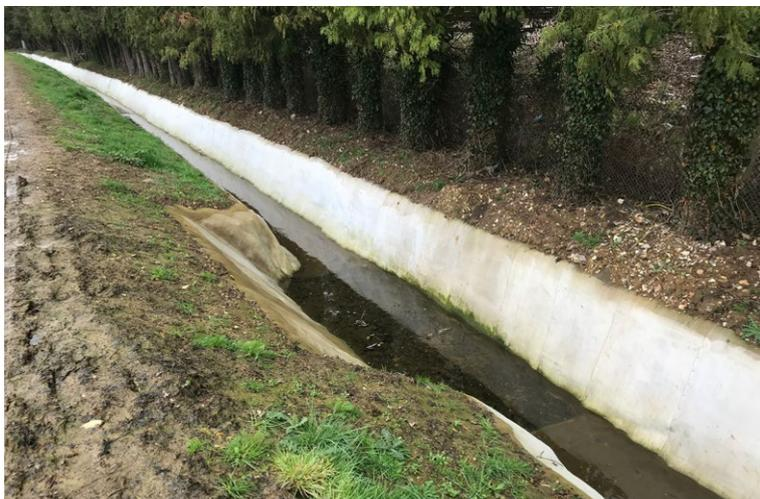
*Sump area lined with CC13<sup>™</sup> in a CC8<sup>™</sup> channel*
