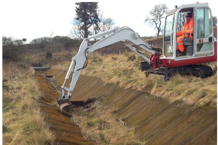
*Excavator with rubber tipped blade used to clear silt trap*
