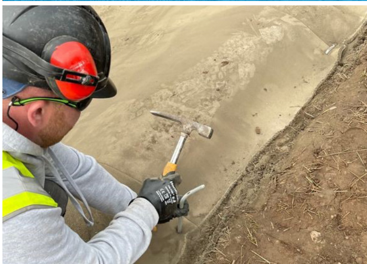
Fixing into anchor trench
