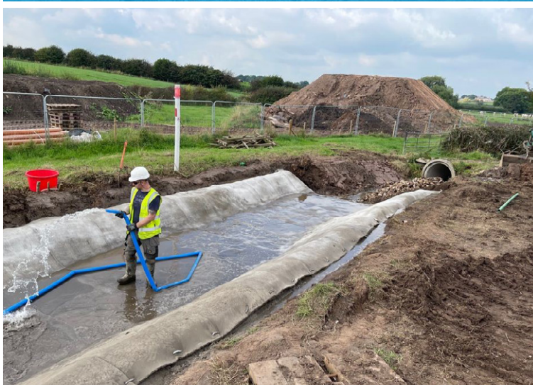
Hydration of finished installation
