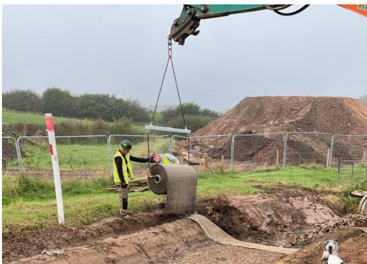
Delivered on Bulk Rolls and deployed from a spreader beam
