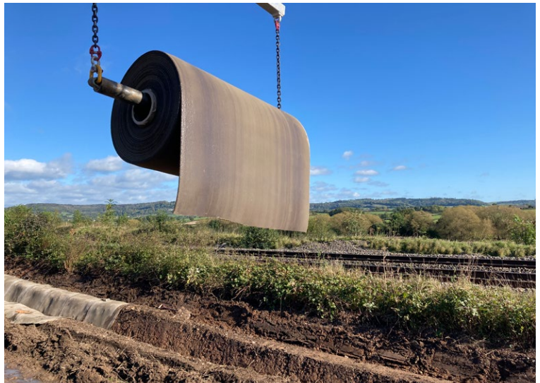
Bulk Rolls dispensed from a spreader beam
