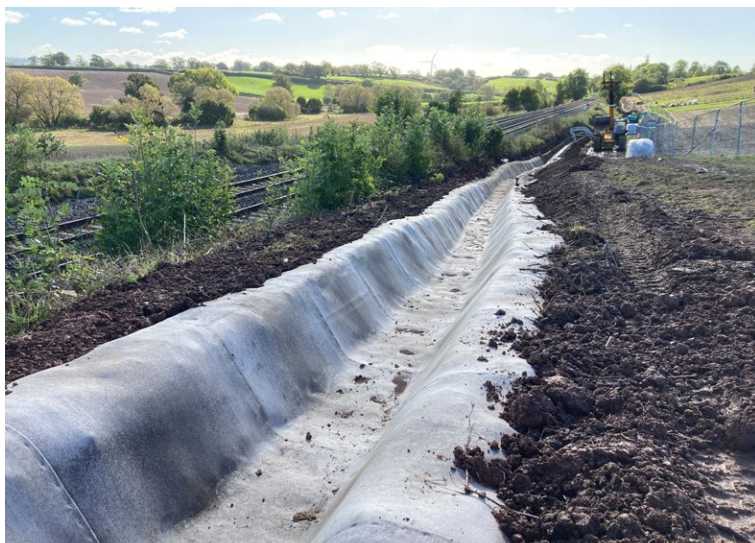
Installed and hydrated CC
