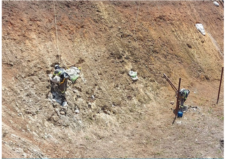
Contractors filling slope irregularities with sand-cement bags
