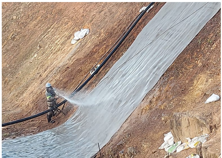
CC5™ hydrated with the use of a hose
