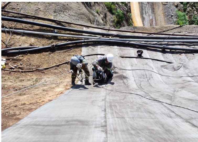
CC5™ overlaps secured with sealant and 25mm screws
