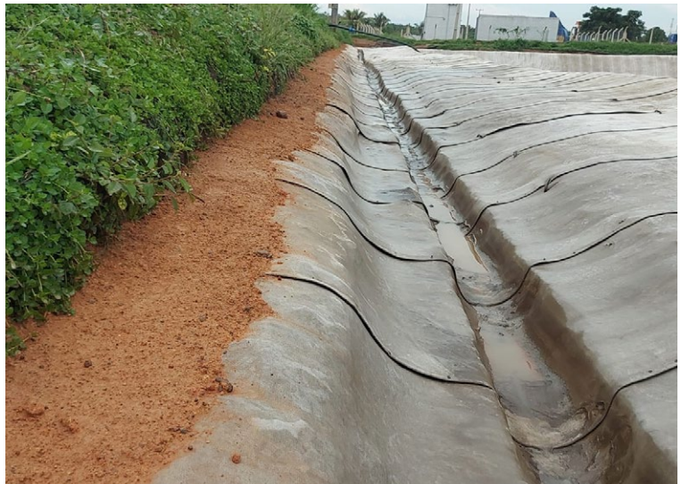
A crest drainage channel was formed in CC and the anchor trench back filled with soil
