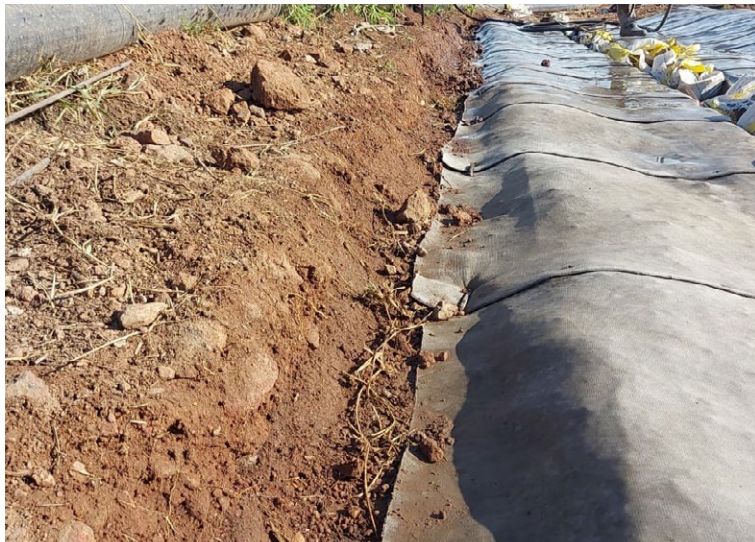
CC5™ secured with 500mm steel pegs at the base of the anchor trench
