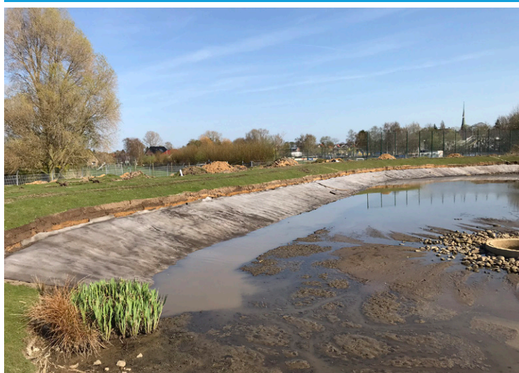
Completed installation prior to placement of clay top cover
