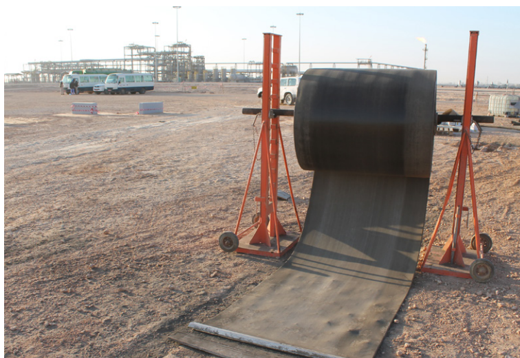
CC was batched and moved to site by hand
