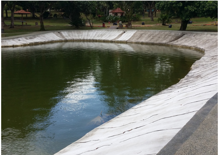
CC was able to accomodate curved sections of slope
