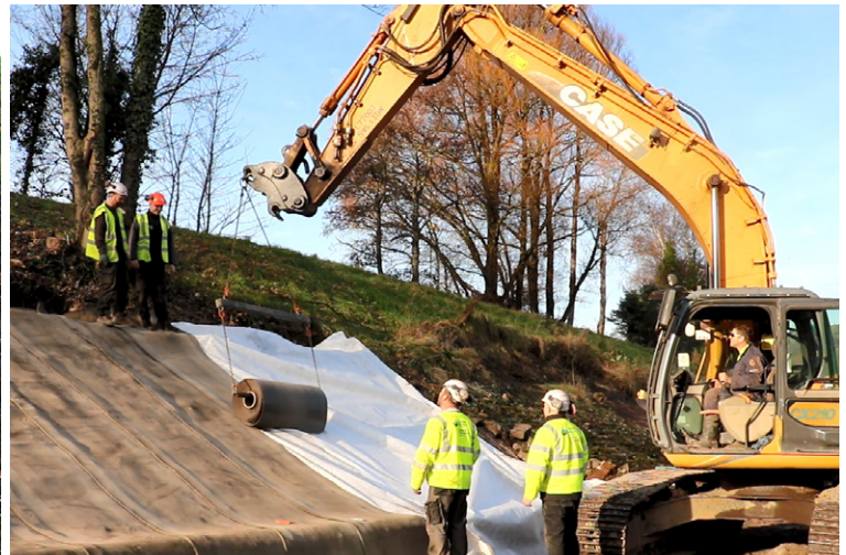
Dispensing of bulk roll CC13 via spreader beam
