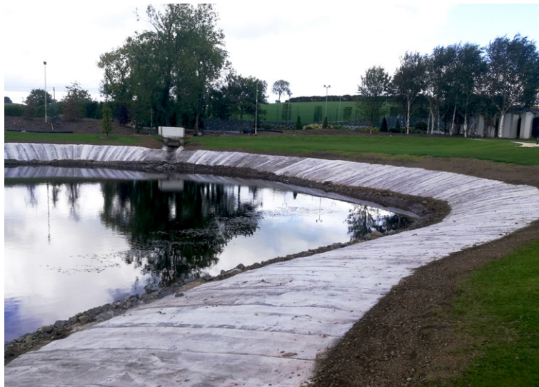
Anchor trenches backfilled and compacted
