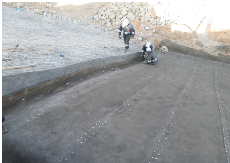
CC secured with ground pegs and jointed using screws
