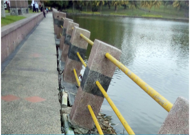
Guard rails collapsing into lake due to erosion
