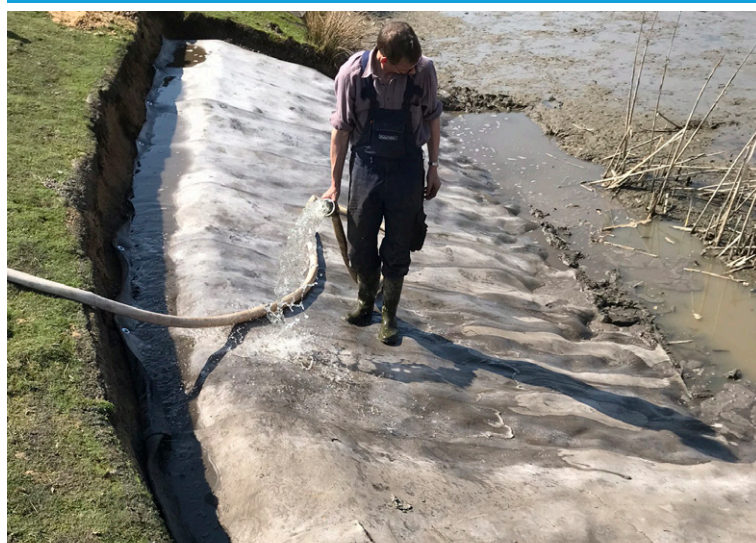
Platipus ground anchors fixed the CC to the substrate at the toe
