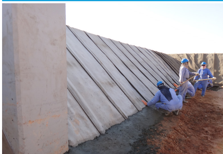
Applying concrete backfill to anchor trenches post-hydration
