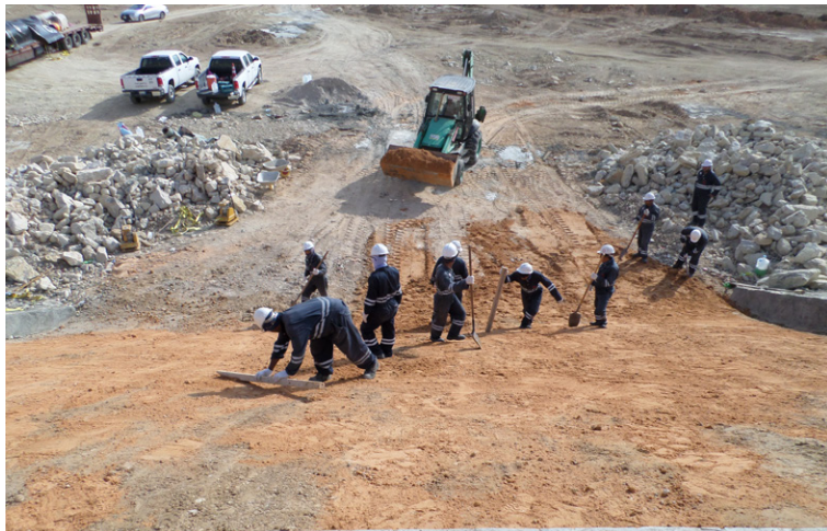
Levelling and backfilling the substrate following compacting
