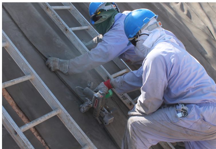
Thermally bonding CC joints
