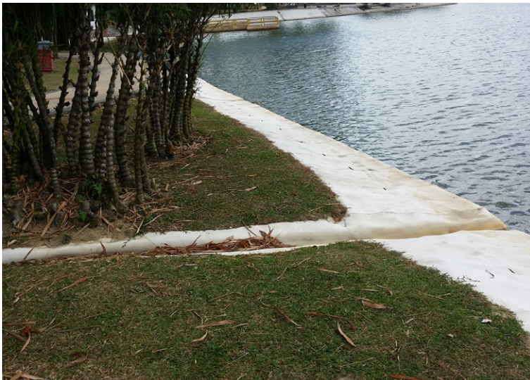
CC buried in anchor trenches to preserve grassy areas above slope
