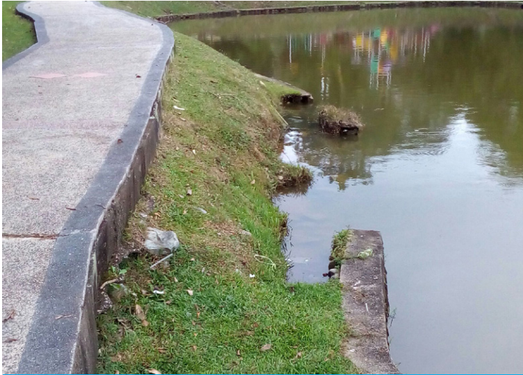
Sections where erosion has caused the soil slope to collapse into the lake
