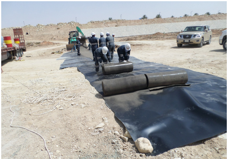
Batched lengths of CC ready for transportation to site
