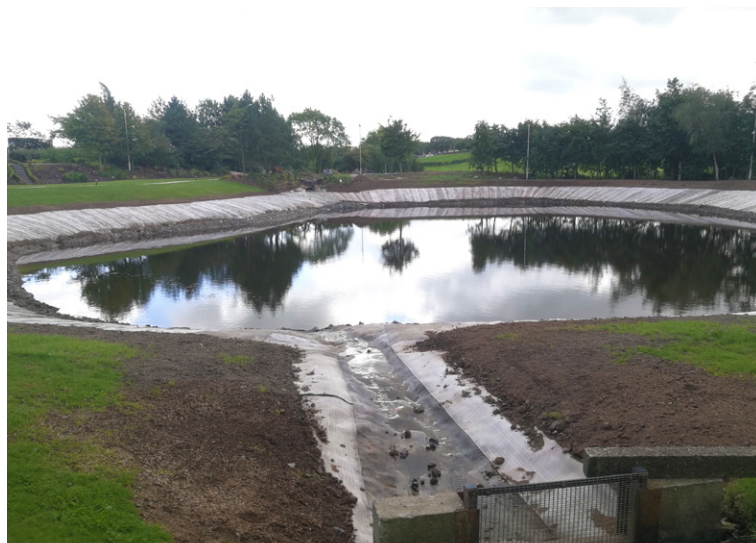
CC lined pond inlet channel
