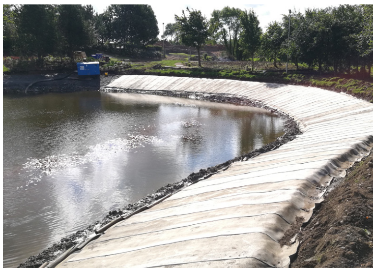
CC secured into crest and toe anchor trenches
