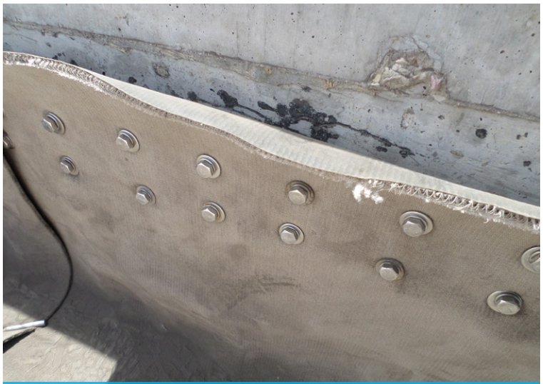
CC fixed to existing concrete at crest using steel bolts
