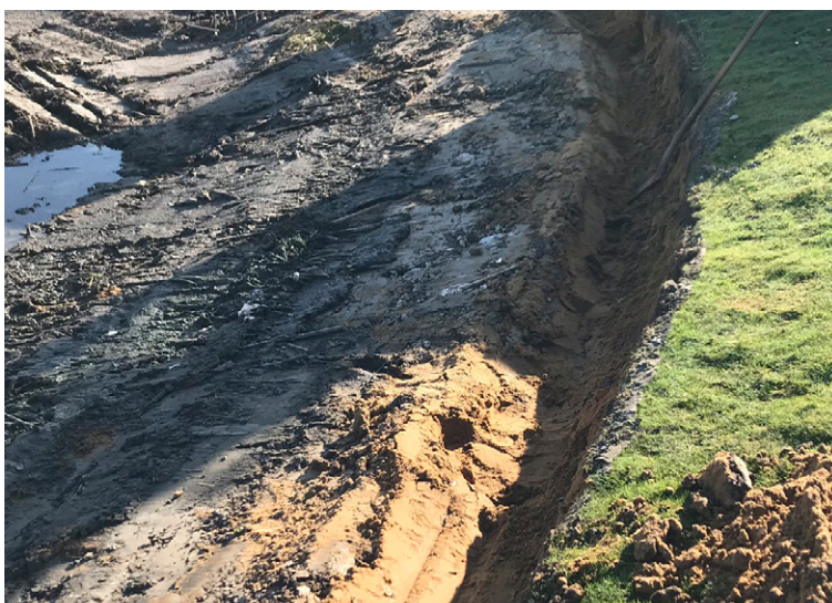
Clay topsoil removed using a digger & an anchor trench was created manually
