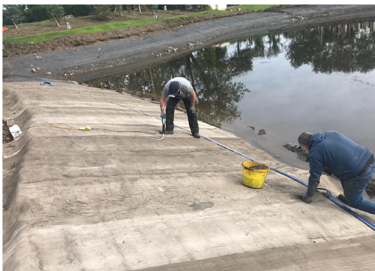
CC overlaps jointed using screws, placed at 200mm intervals
