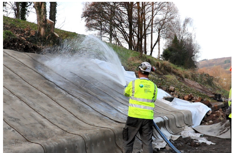
Hydration of the CC lined sections using water from the River Taff
