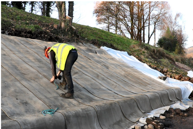
Fixing of the overlapped CC layers using SS screws at 150mm centres
