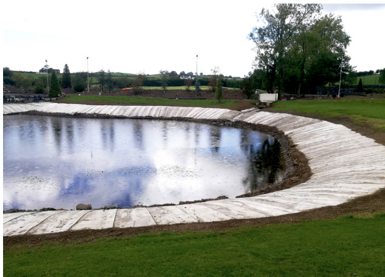
Inlet channel and completed CC installation
