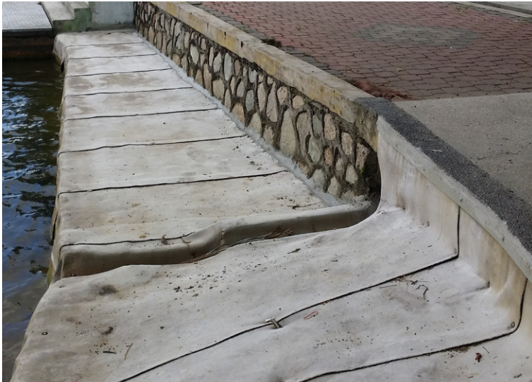
Ground pegs, wall plugs, screws & poured concrete used to joint & fix CC
