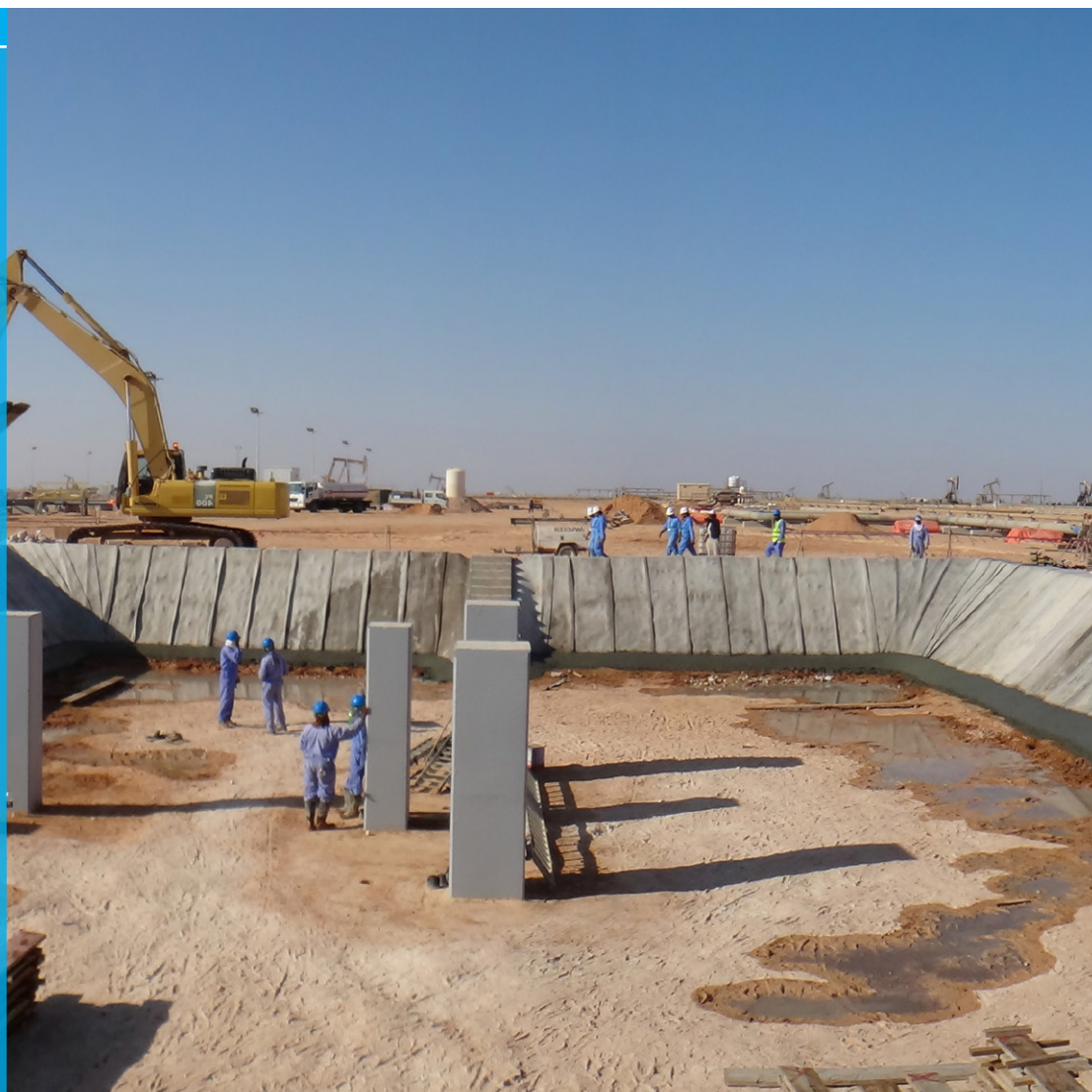
Completed, lined blow down pit
