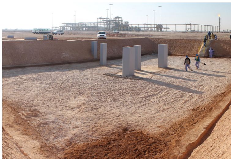
Excavated pit prior to lining
