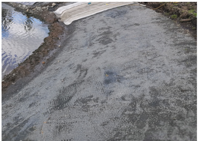
Crushed gravel compacted on slope for optimum substrate
