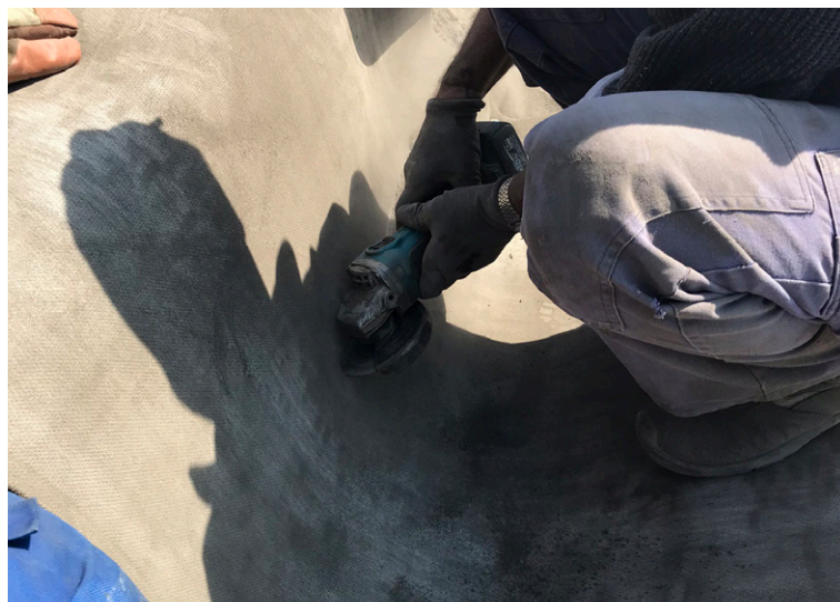
A disc cutter was used to cut the CC to length
