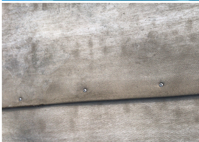
Overlapped layers were jointed using stainless steel screws
