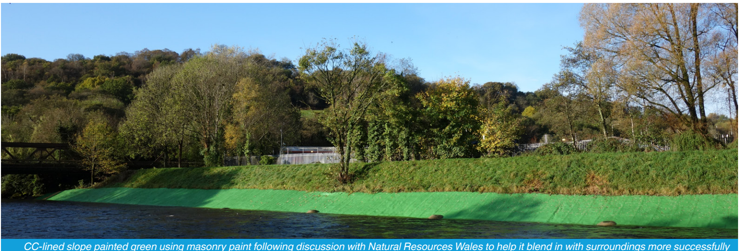
CC-lined slope painted green using masonry paint following discussion with Natural Resources Wales to help it blend in with surroundings more successfully
