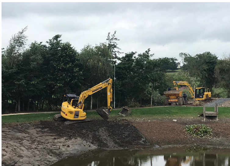
Excavation of embankment
