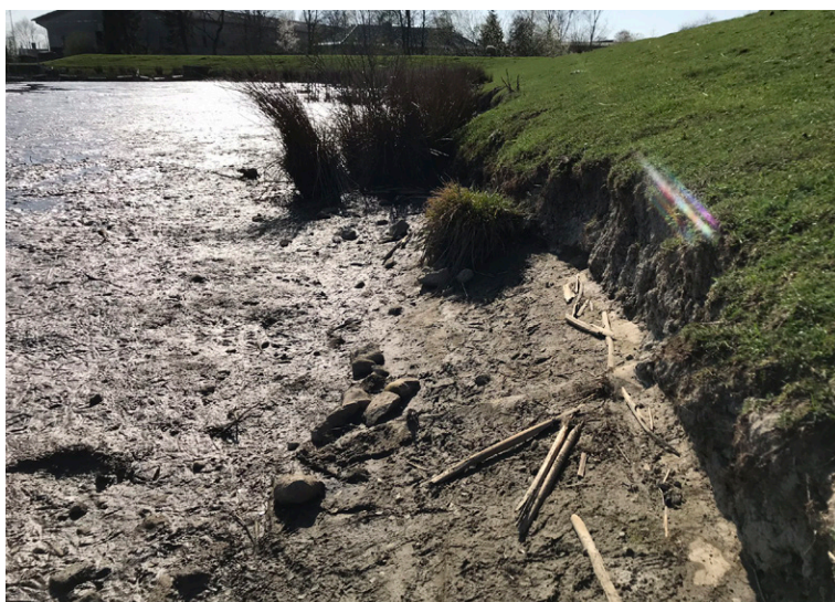
Section of embankment affected by erosion
