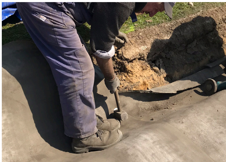
Ground pegs were used to secure CC at the crest
