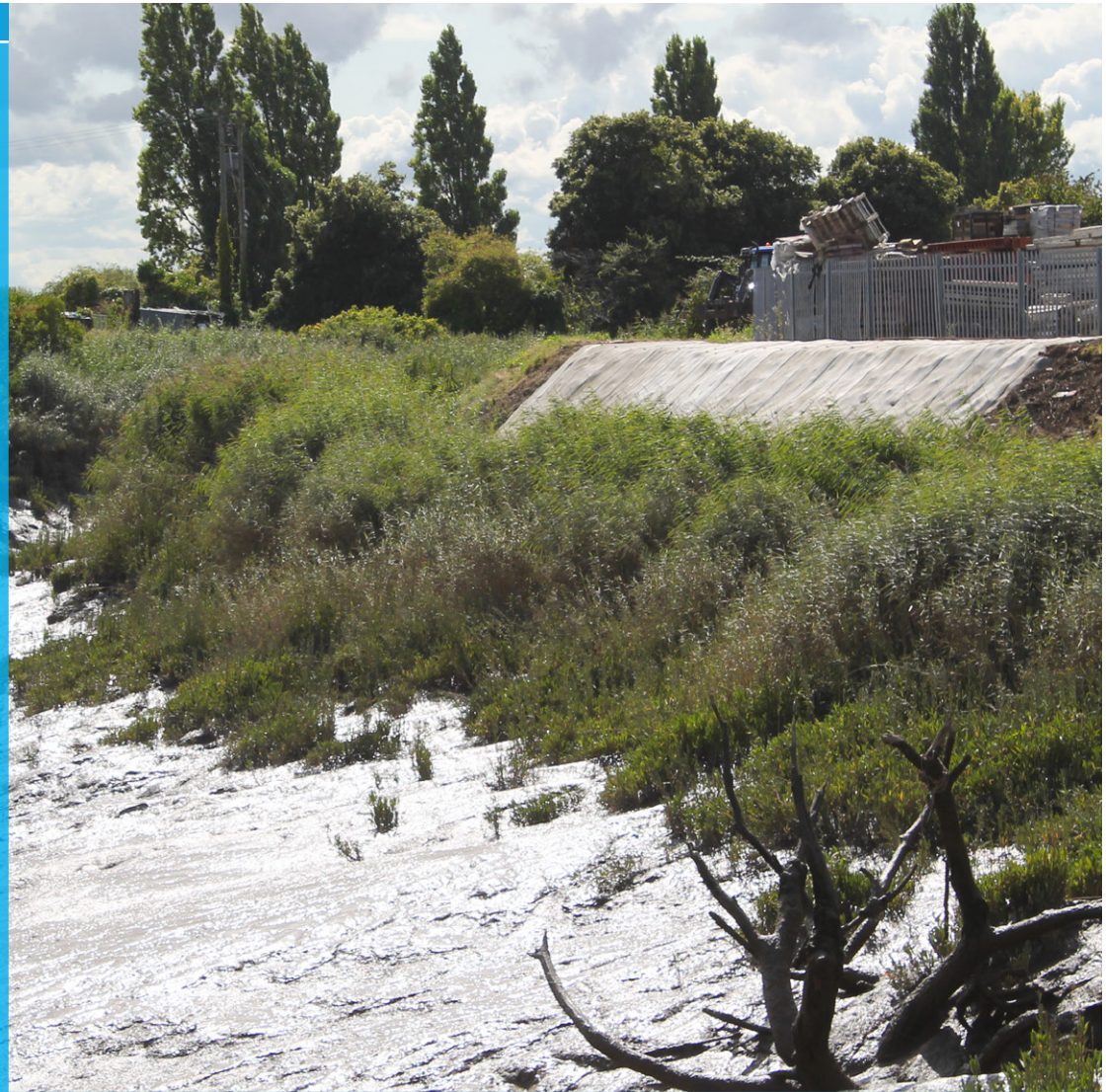
Completed first section of lined berm
