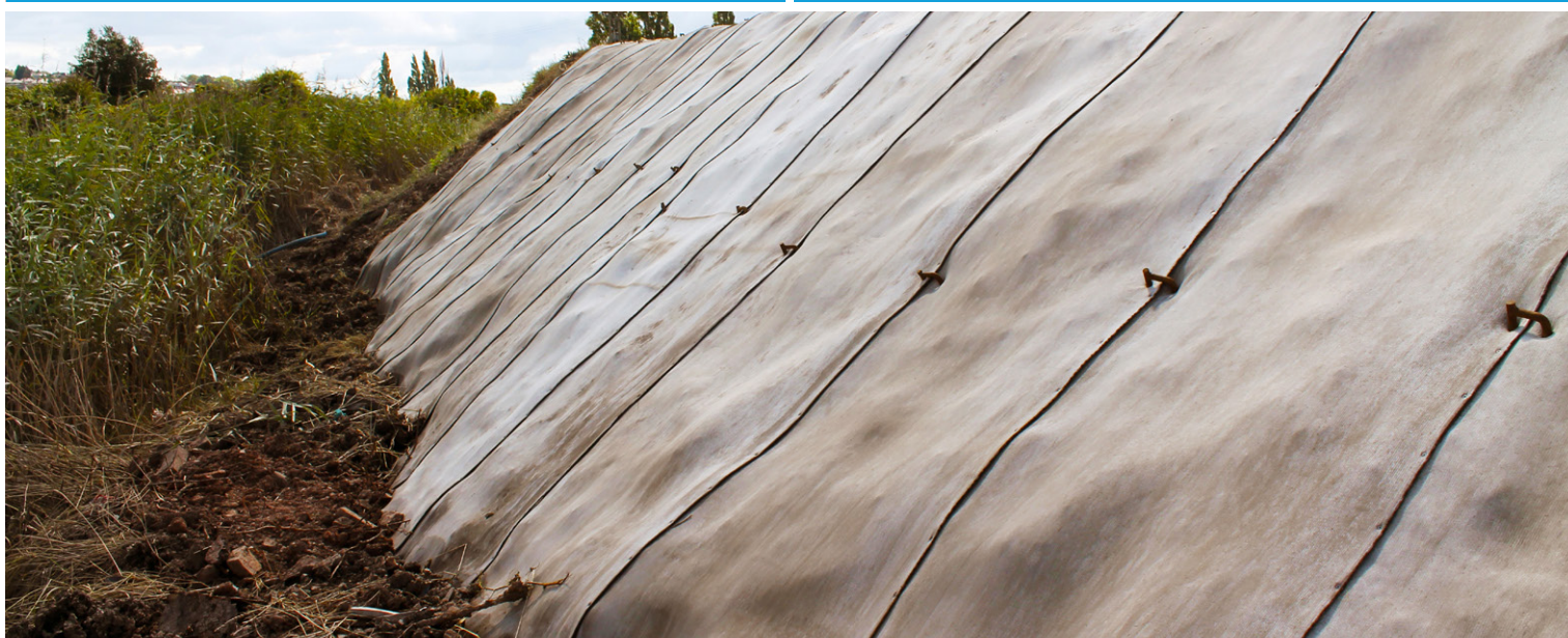
Completed first section showing toe anchor trenching, screw fixings and ground peg placement
