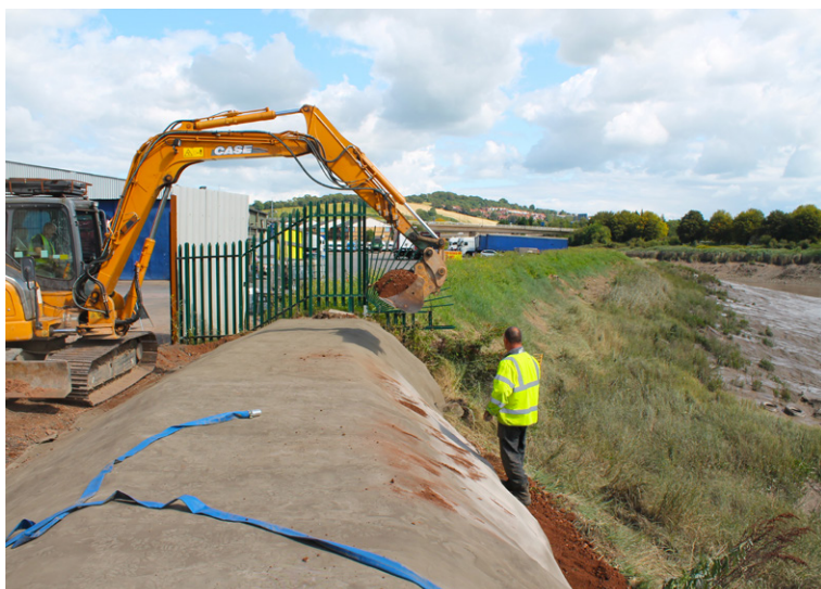
Backfilling anchor trench at toe of second section berm
