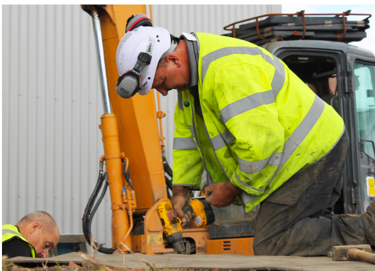
Fixing of the CC overlaps with stainless screws at 150mm centres
