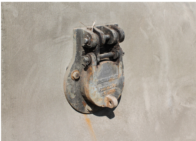
Drain pipe cover access through CC
