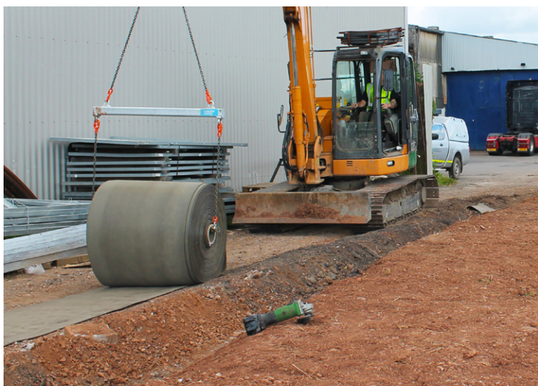
Batching lengths of CC from spreader beam suspended bulk roll
