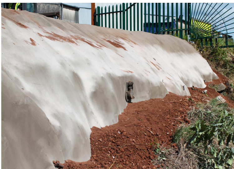
Backfilled anchor trench post hydration
