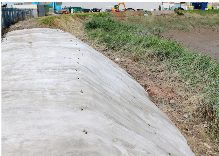
Completed first section, showing ground pegs at 3m intervals
