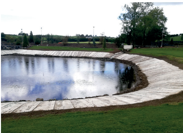
Inlet channel and completed CC installation
