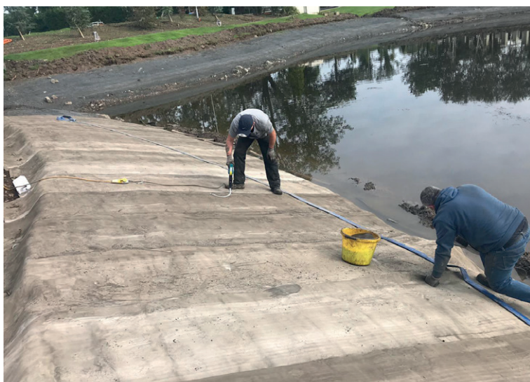
CC overlaps jointed using screws, placed at 200mm intervals
