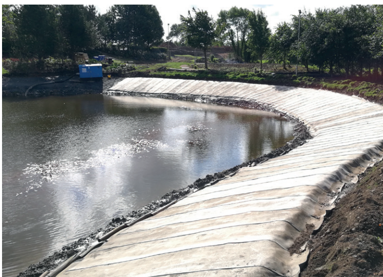
CC secured into crest and toe anchor trenches
