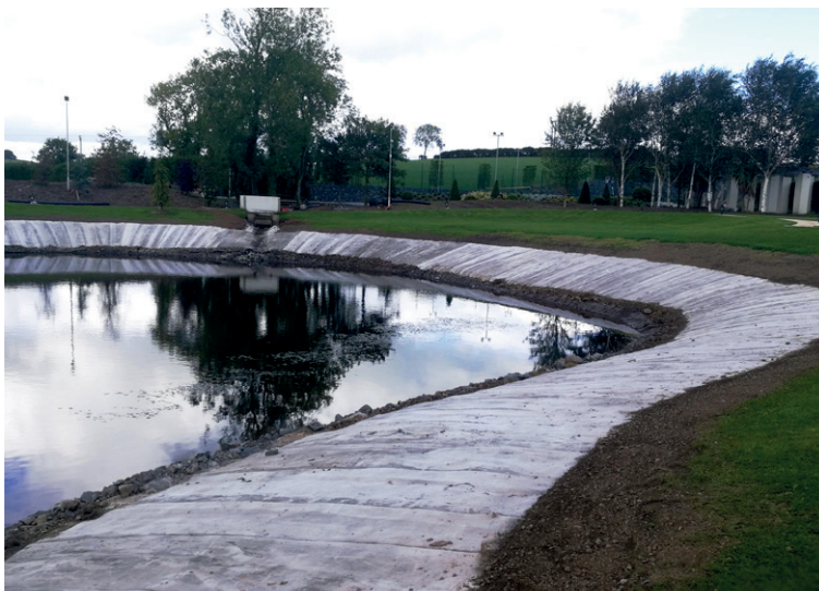
Anchor trenches backfilled and compacted
