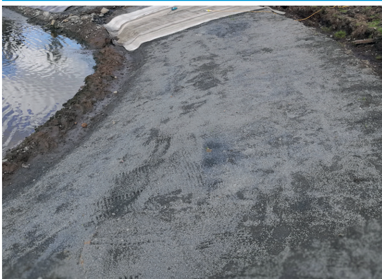
Crushed gravel compacted on slope for optimum substrate
