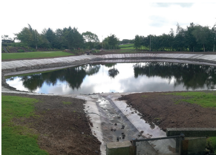
CC lined pond inlet channel
