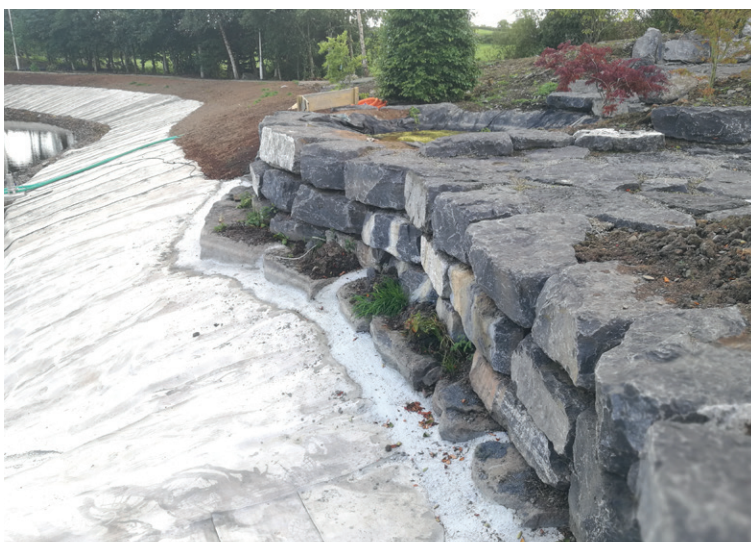
Concrete fillet applied at CC and rock termination
