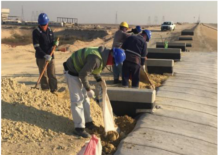
Anchor trenches backfilled to prevent ingress below material
