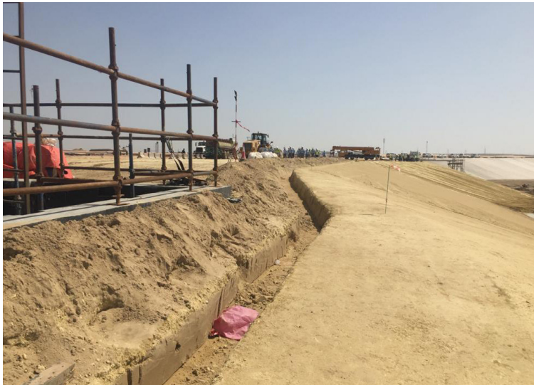
Anchor trenches were created prior to installation
