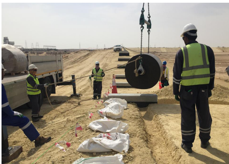
CC bulk rolls deployed from slope crest
