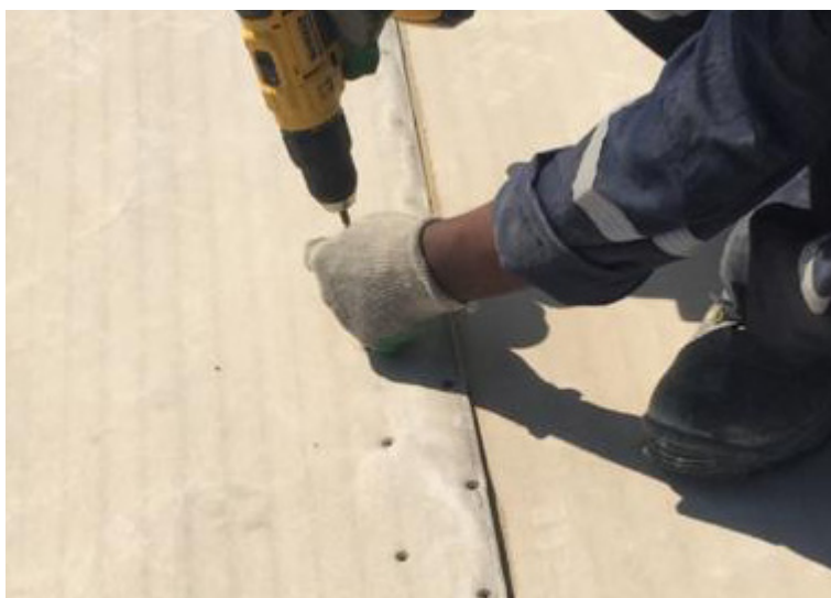
Screws inserted in a zig zag pattern to joint overlaps
