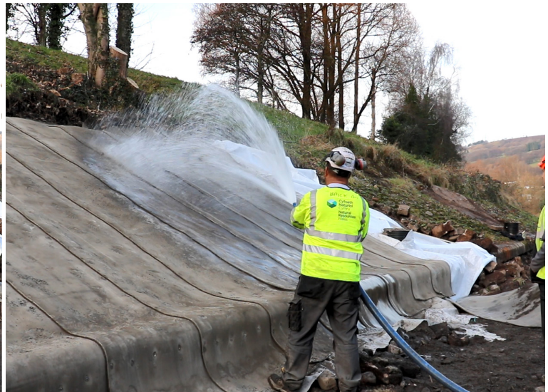
Hydration of the CC lined sections using water from the River Taff
