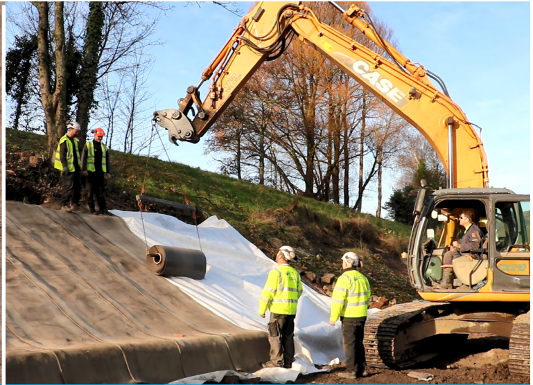
Dispensing of bulk roll CC13 via spreader beam.
