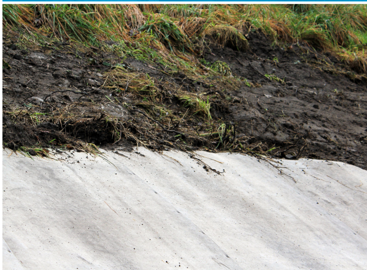
Anchor trenching of the CC13 midway up the embankment.
