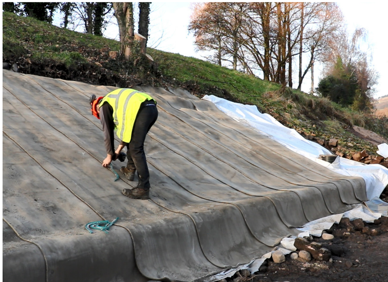
Fixing of the overlapped CC layers using SS screws at 150mm centres
