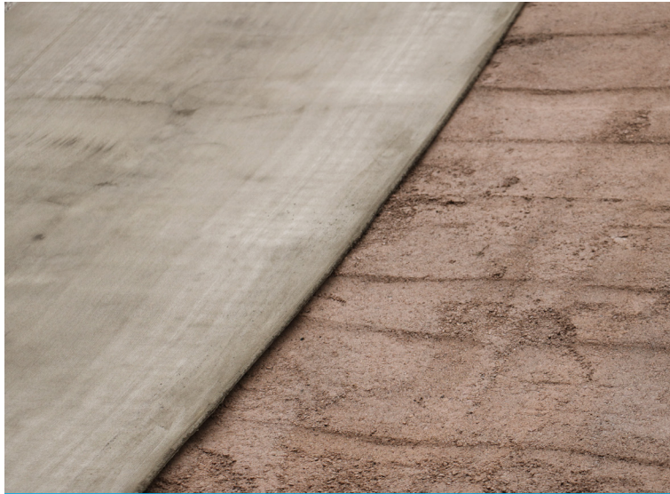
Preparation of the slope; regrading and placing of the geotextile
