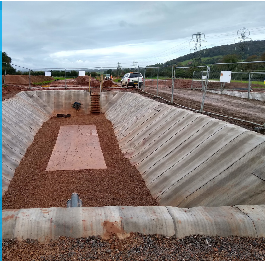
Completed bank erosion protection installation in Somerset
