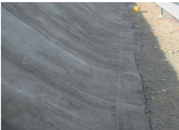
Pegging at toe of slope
