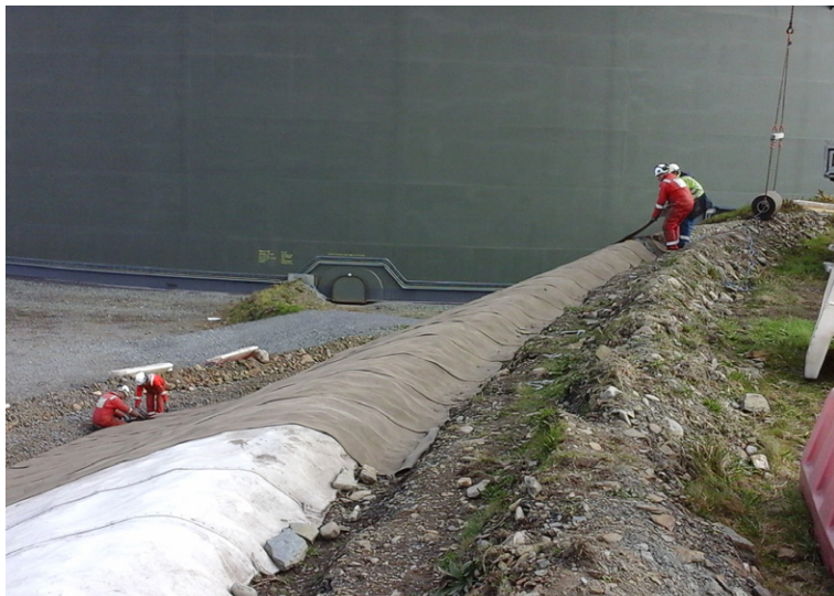
Crest anchor trench detail
