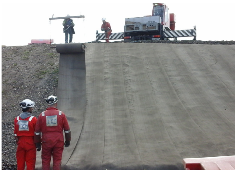
CC secured in toe anchor trench and unrolled up bund height
