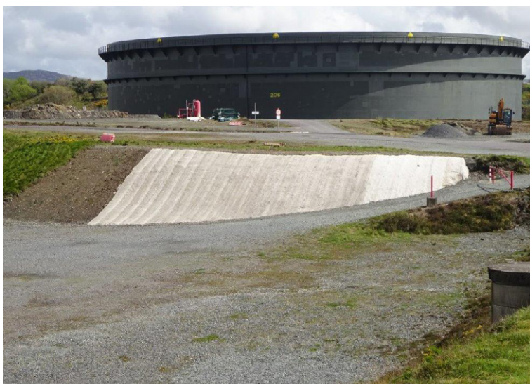
CC bund installation completed
