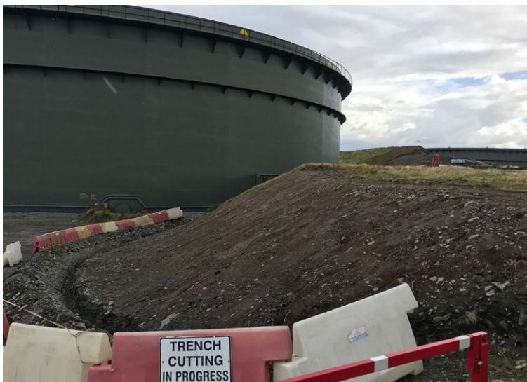
Bund following grading ready for installation
