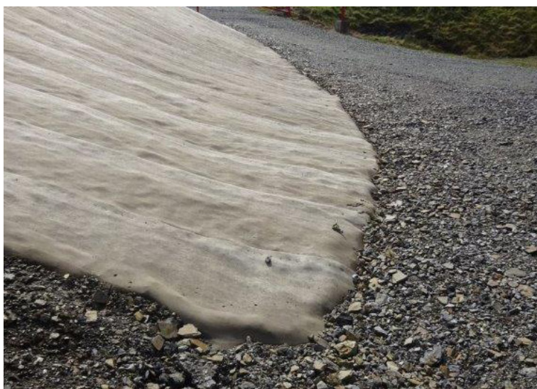
Anchor trenches backfilled following hydration
