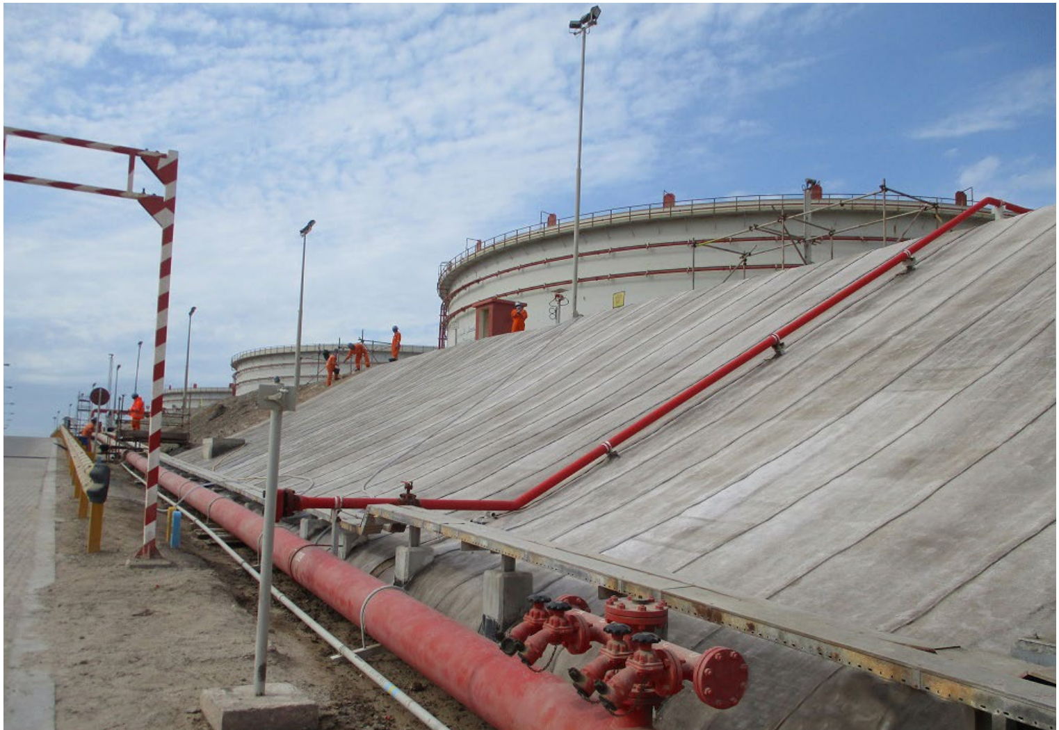
Completed phase of installation
