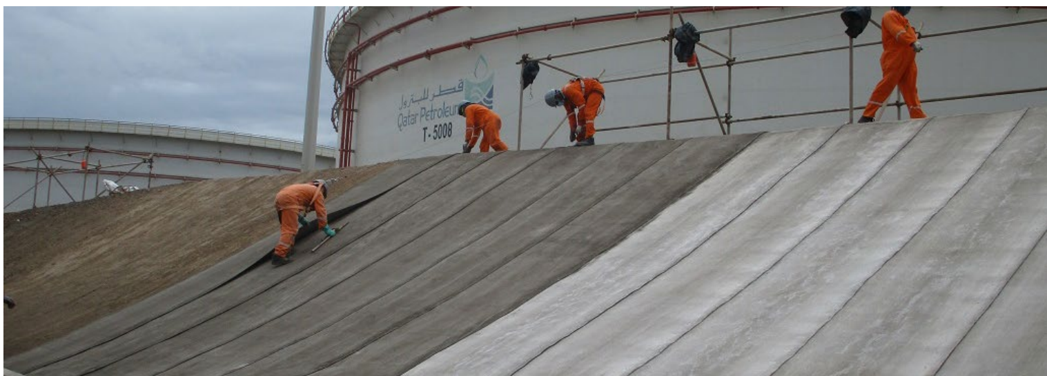
CC8™ installed vertically down the bund
