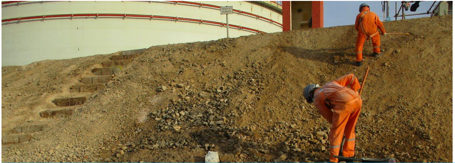
Bund being prepared before installation works
