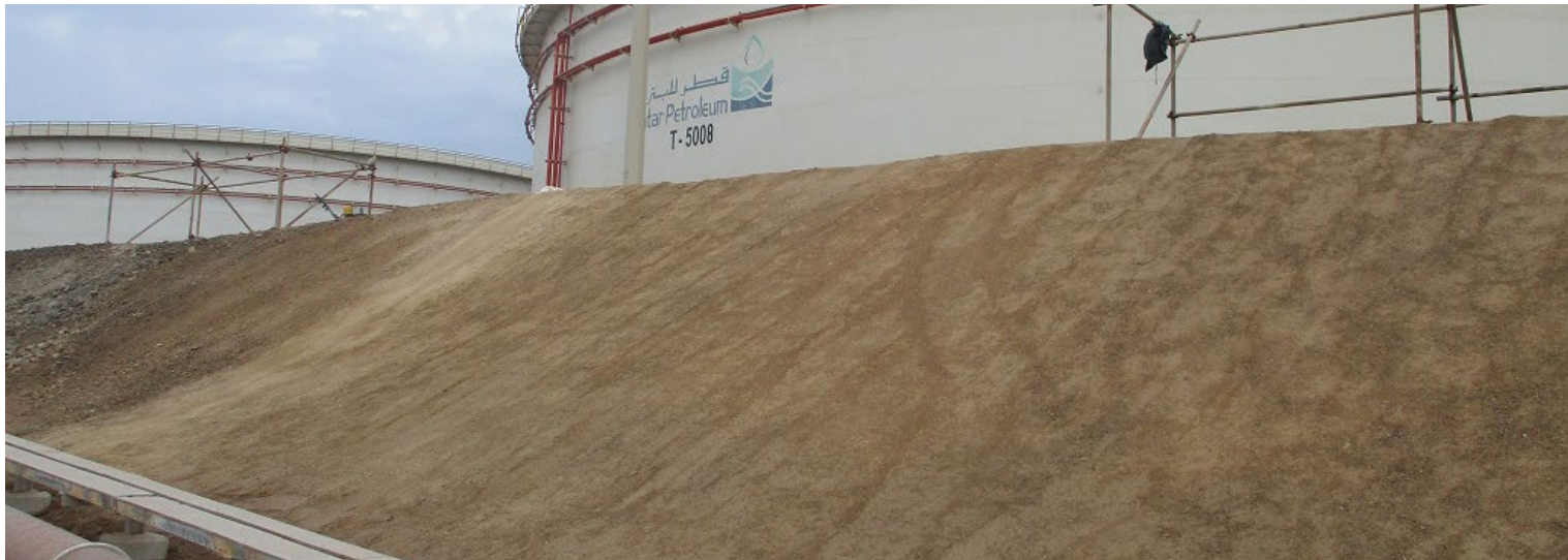
All protrusions and voids removed
