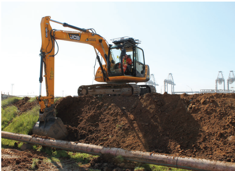
The bunds were excavated to prepare them for installation
