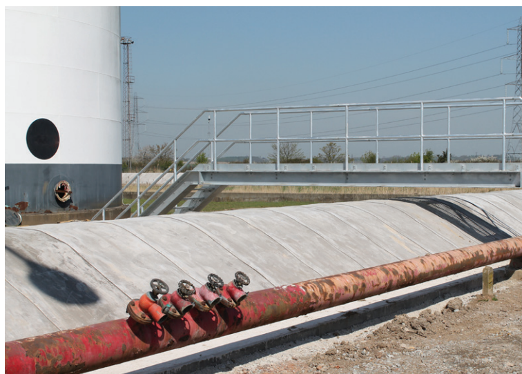
CC easily accommodated existing pipework
