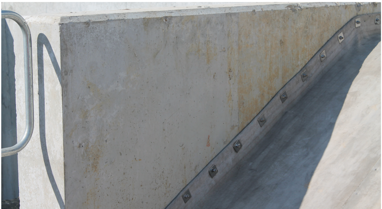
Headwall termination detail
