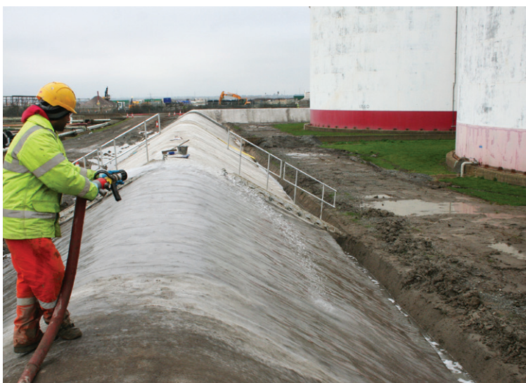
Hydration of CC from on site mains water supply
