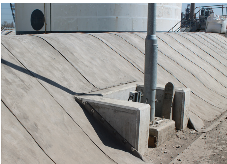
CC termination at a headwall
