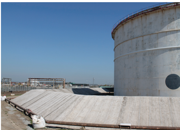
CC can easily be fitted around corner details of bunds
