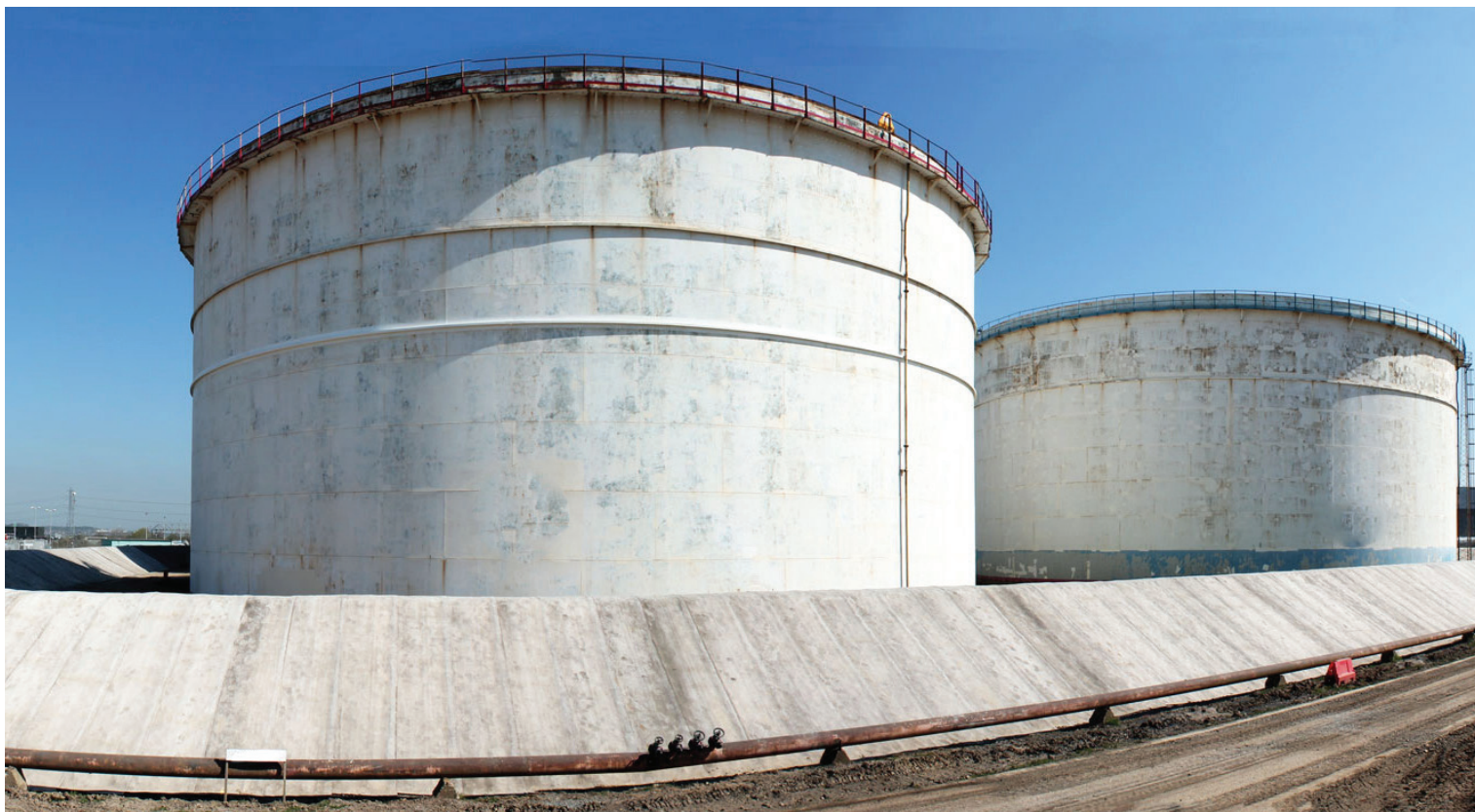
An completed section of bund next to two storage tanks
