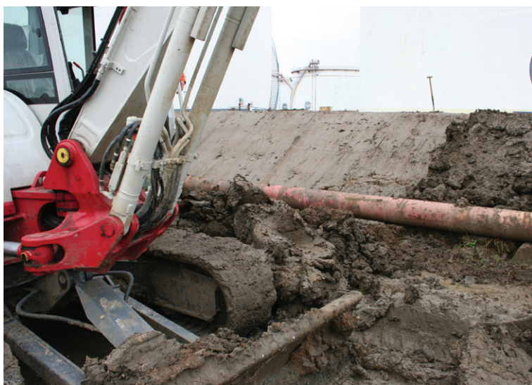
Preparation/ grading of the clay bund
