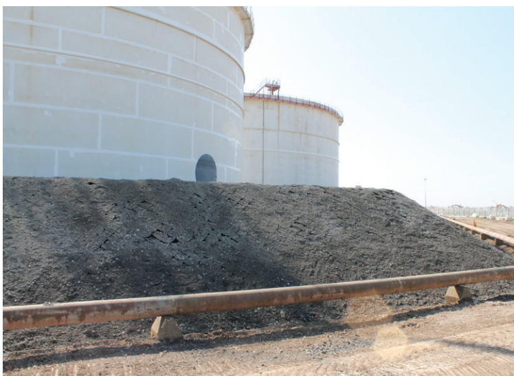
The graded bund ready for installation
