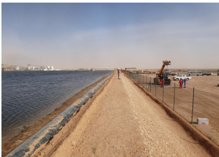
The bund was graded prior to installation
