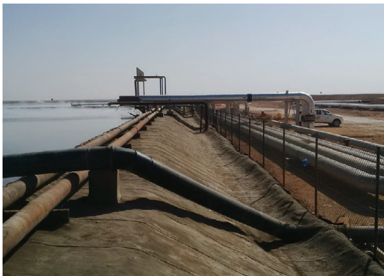
The CC edges were buried in pre-dug anchor trenches
