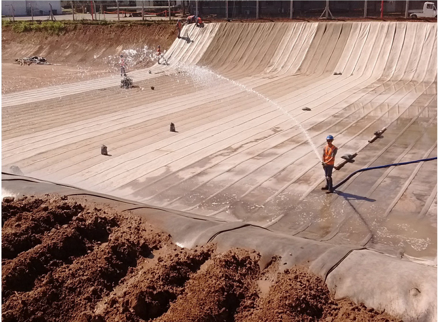
A total of over 20,000m 2 of CC were installed
