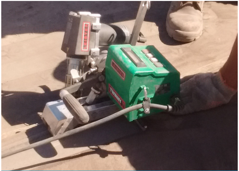
Layers of CC thermally bonded to reduce joint permeability
