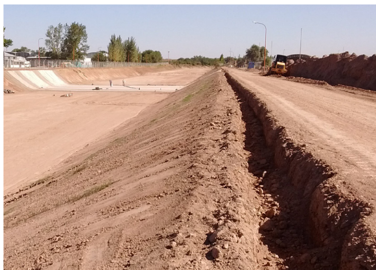
Canal section following ground works and preparation of anchor trenches
