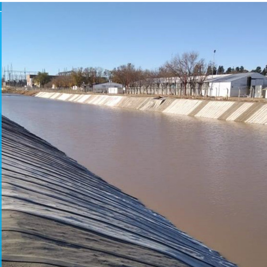
Completed CC canal lining installation
