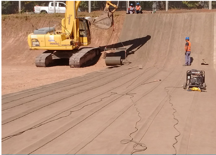
CC bulk rolls deployed from spreader beam and excavator
