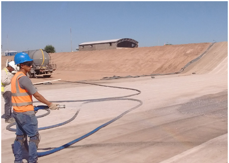
CC hydrated using bowser and hose
