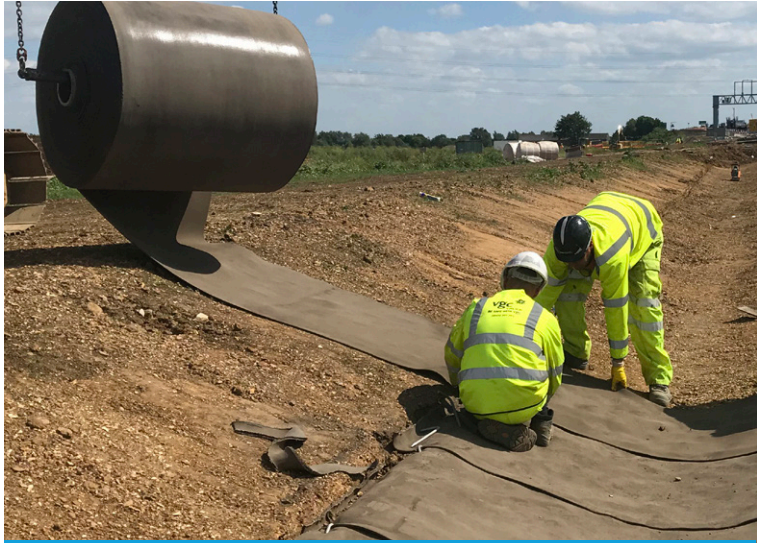
Deployment of CC and fixing of material in anchor trench
