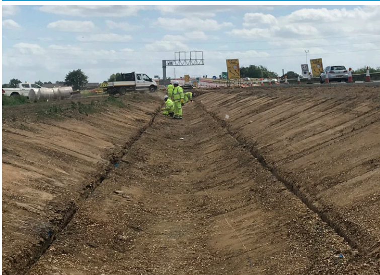
Completed anchor trenches
