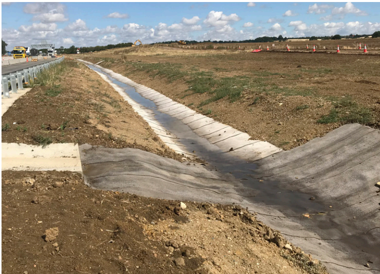
CC extended to full height where slipform drainage enters channel
