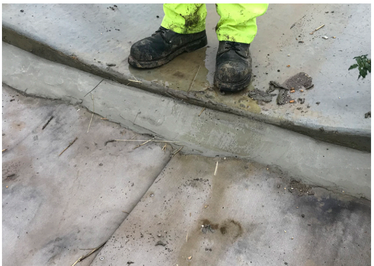
Grout fillet termination
