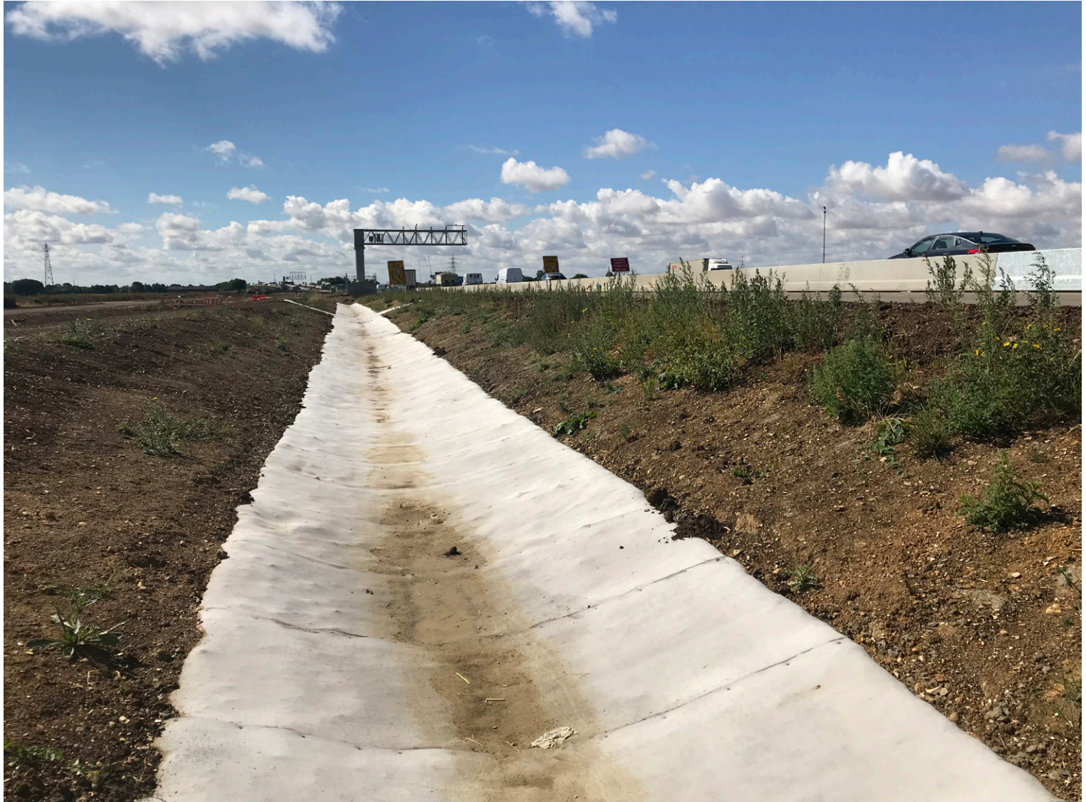
Completed section of CC installation
