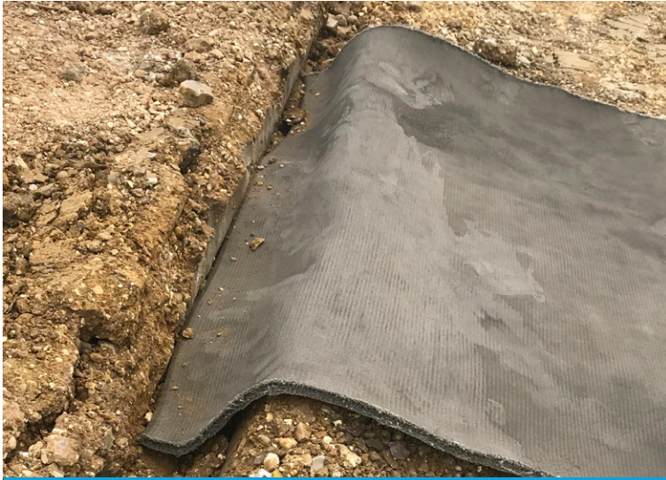
CC laid in anchor trench
