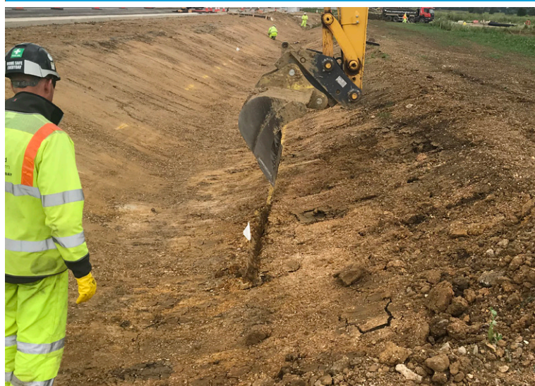
Excavation of anchor trenches
