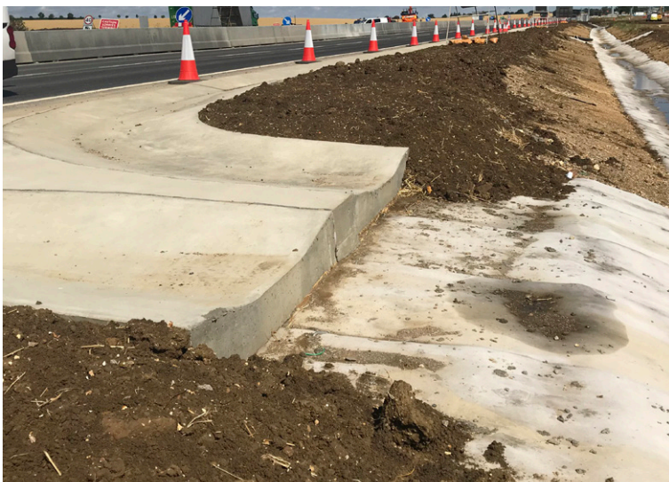
CC to slipform drainage termination
