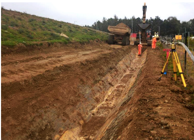
Vegetation and debris removed and the channel excavated for install
