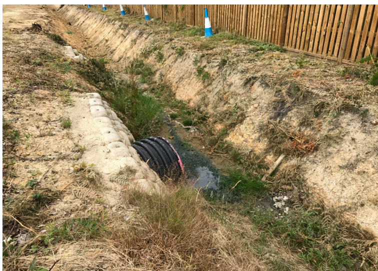
The channel was heavily vegetated, causing blockages and risking flooding
