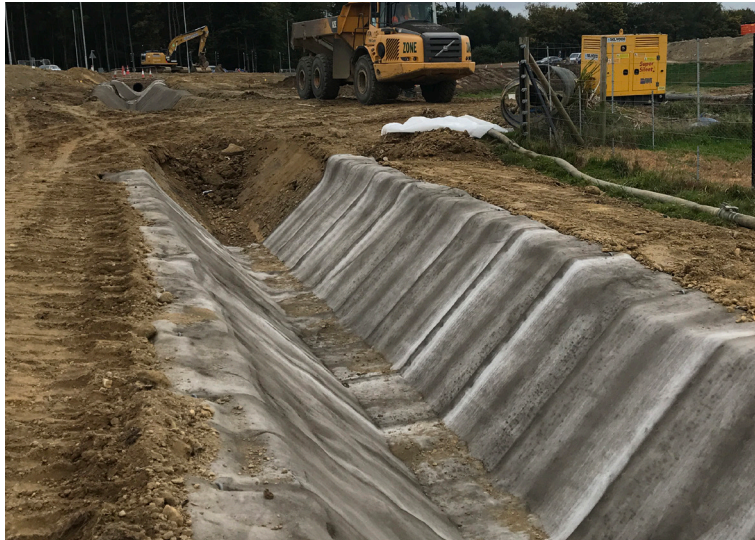
Following hydration, the CC edges were buried in anchor trenches
