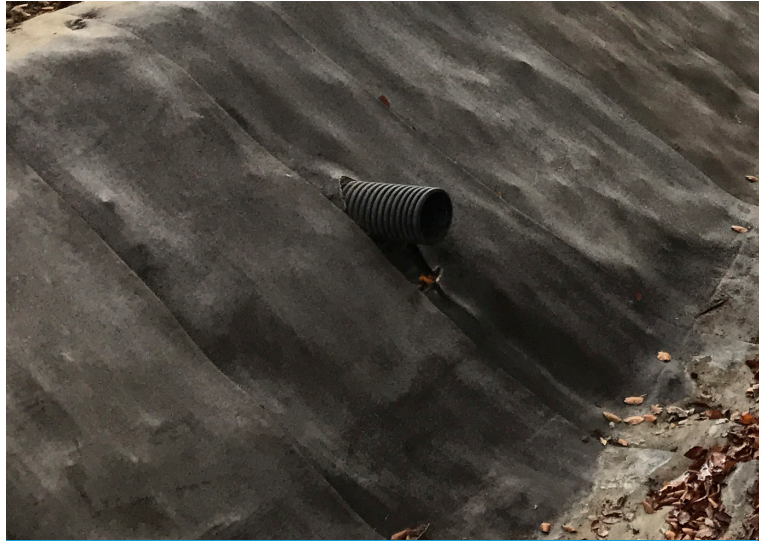
The CC was easily cut to accomodate protruding pipes
