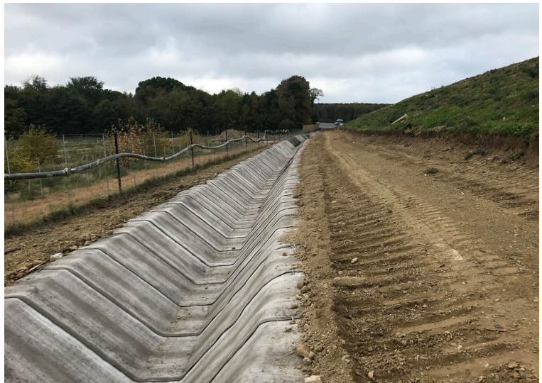
The 360m long channel required 2,165m 2 of CC8™
