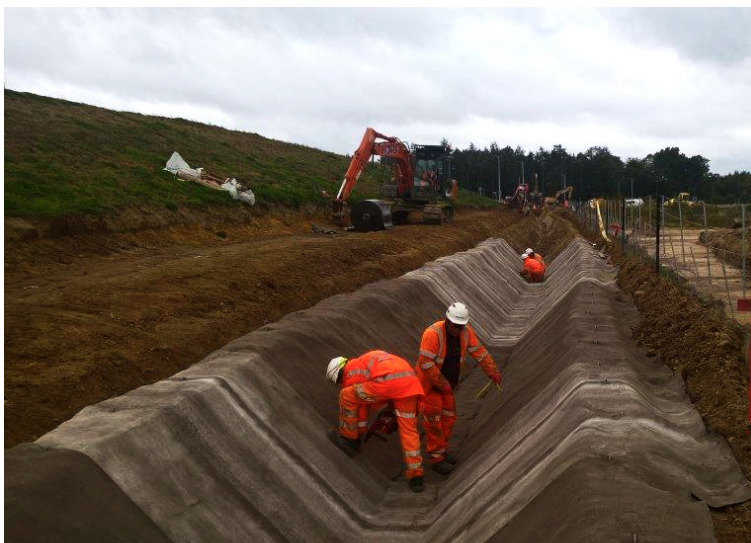
Screws were used to joint the CC overlaps
