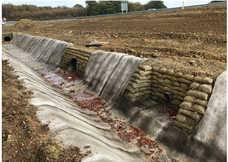
CC installed around headwalls
