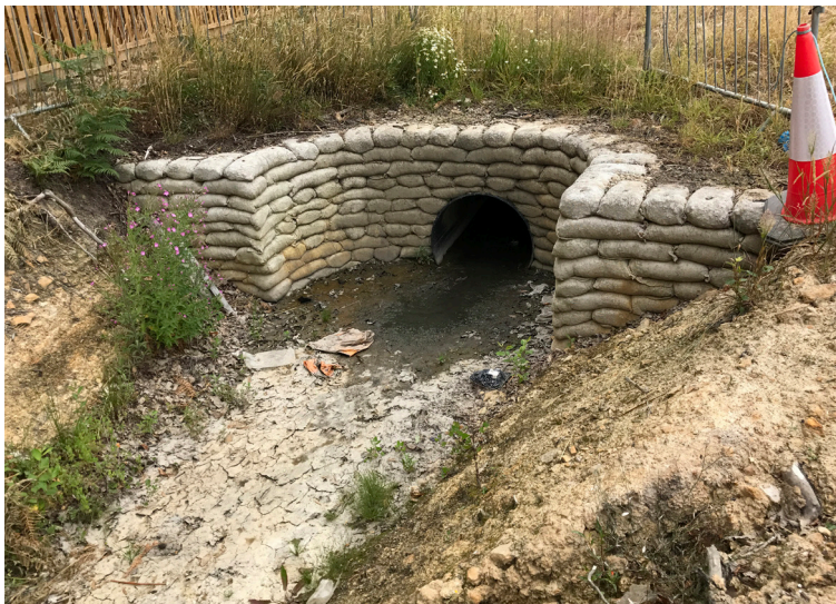
CC was specified as its flexibility could accomodate existing infrastructure
