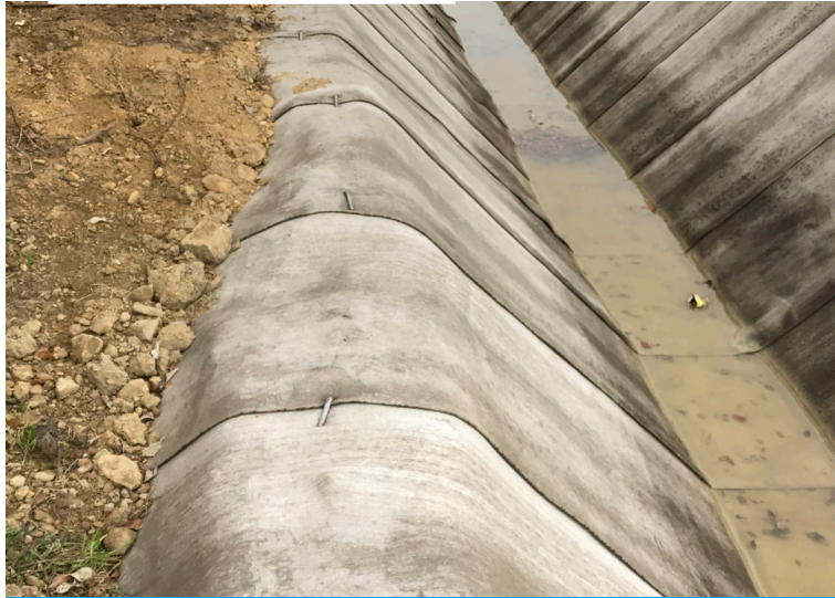
Pegs were used to fix the CC to the substrate
