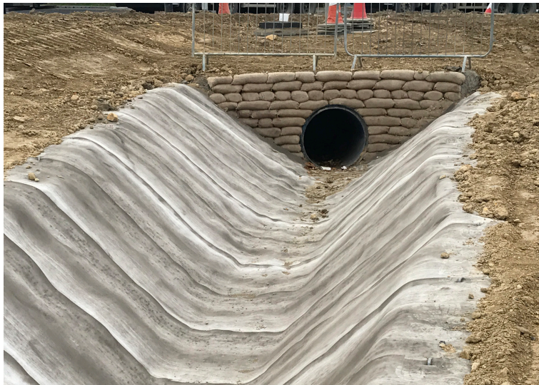
CC ends were sealed with grout around the headwall at the top of the channel
