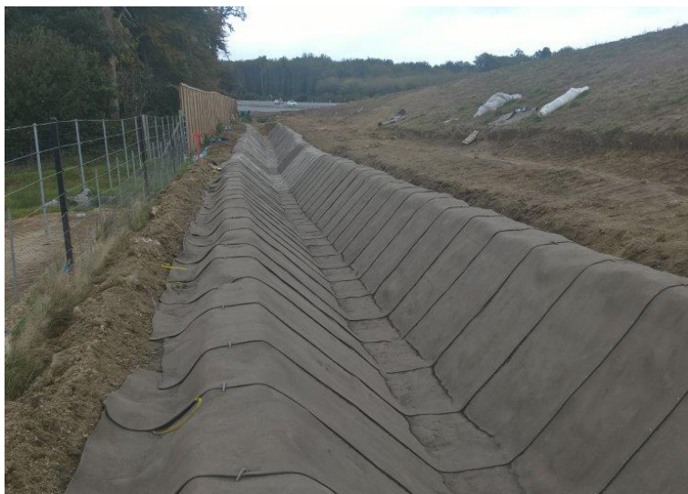
The CC was laid transversely across the channel
