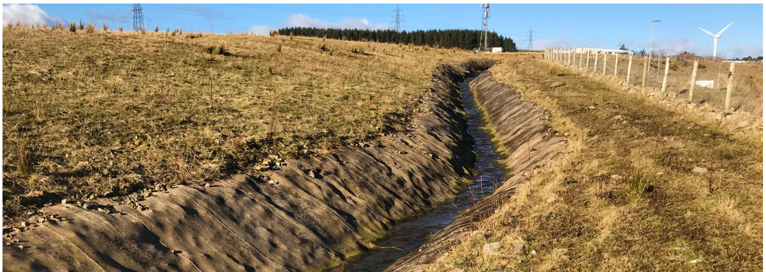
The CC material has blended in with the surrounding environment, whilst the channel is performing hydraulically, exactly as originally designed.
