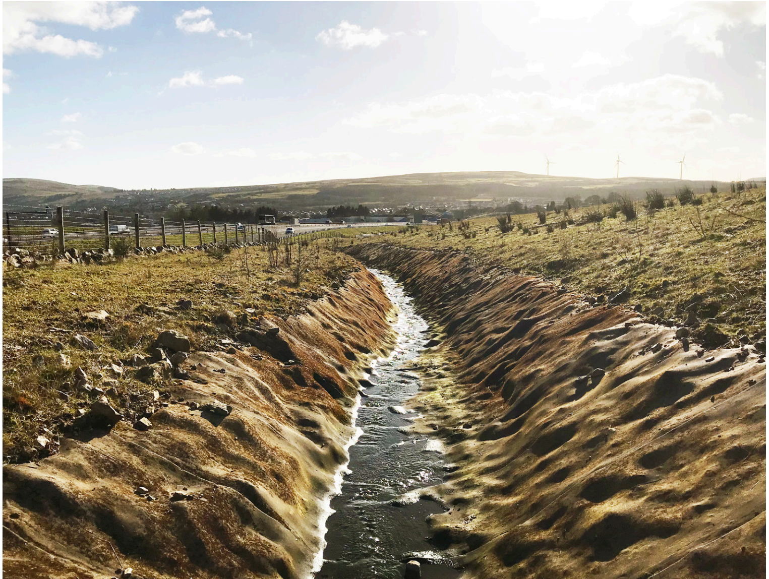
CC lined channel shown five years after installation, having required zero maintenance over that period.
