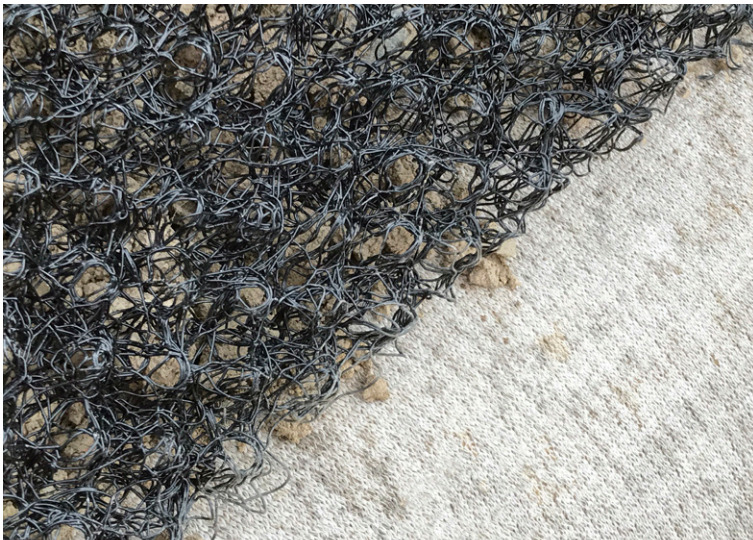
A geotextile was laid to allow vegetation growth over the CC
