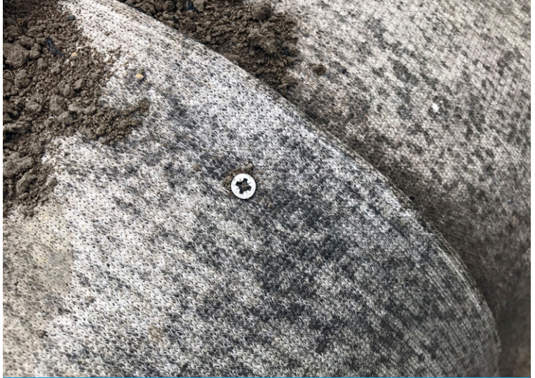
CC was laid transversely and jointed with screws at the overlaps
