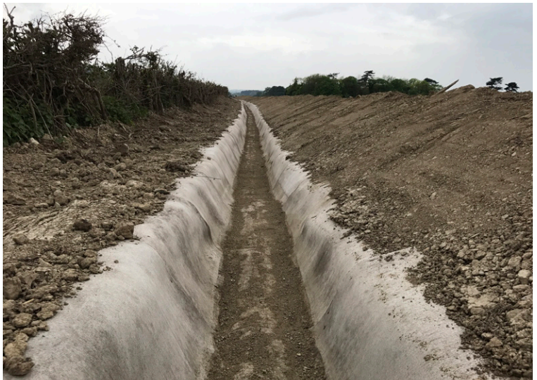
CC edges were captured in backfilled anchor trenches
