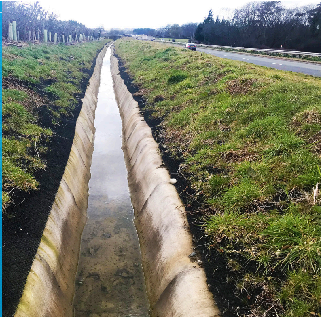
Completed CC lined channel section on the A55, a year after installation.
