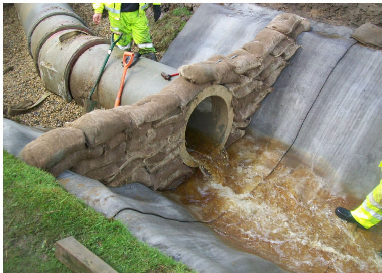
New culvert pipe in place
