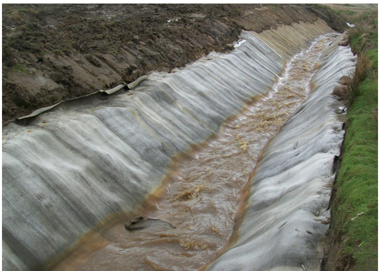
CC laid, prior to backfilling of anchor trenches
