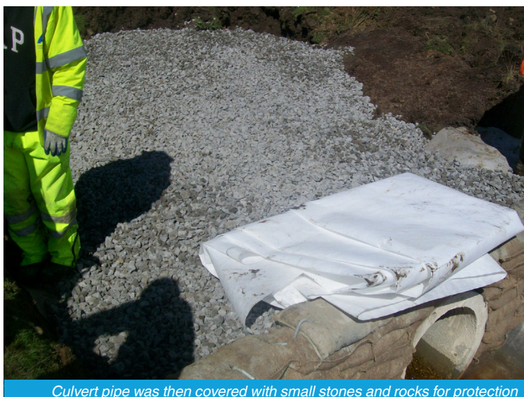
Culvert pipe was then covered with small stones and rocks for protection
