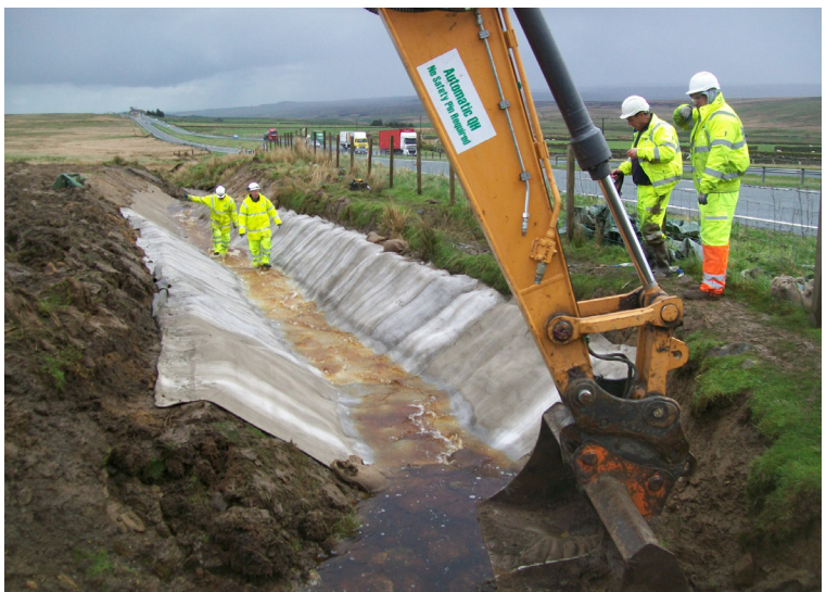
Allowing live water course to hydrate CC
