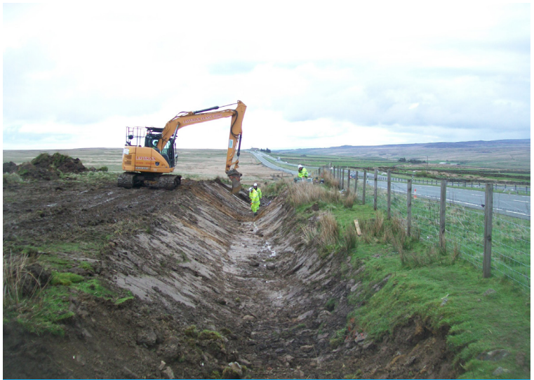
Grading channel profile
