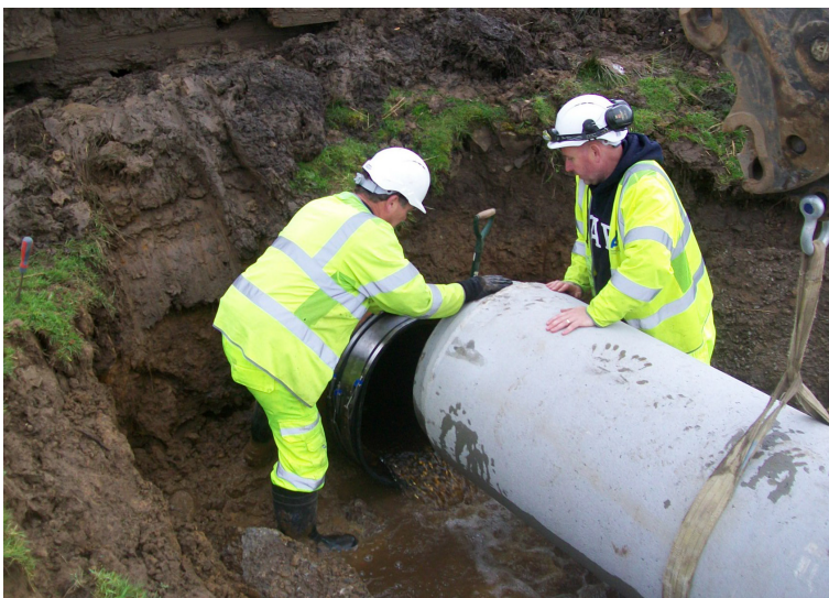
Connecting new pipe to culvert
