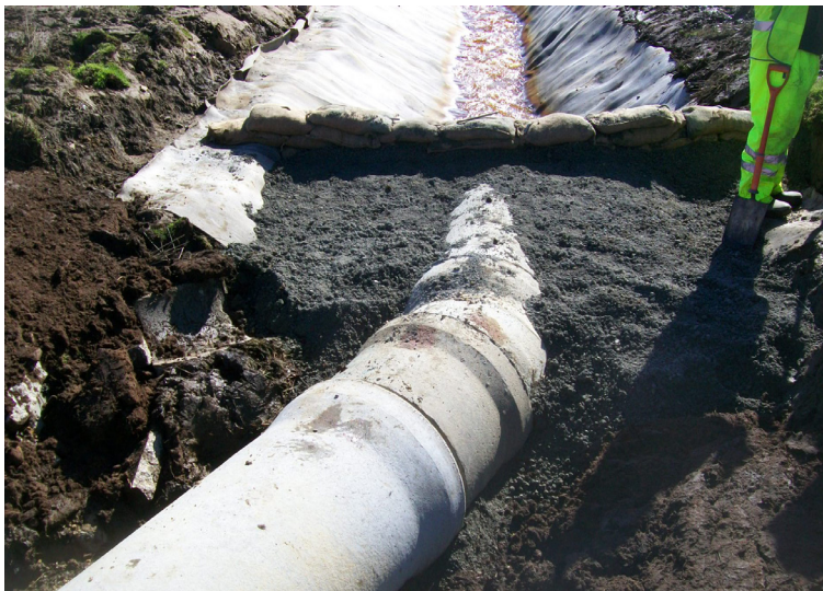
Burying culvert pipe following construction of sandbag wall
