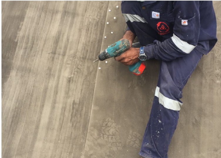
Joining overlaps using stainless steel screws
