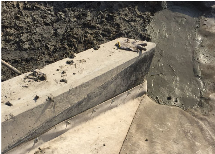
Filling anchor trenches with cement
