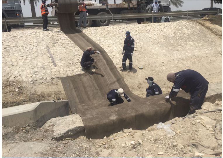
Deployment of CC material
