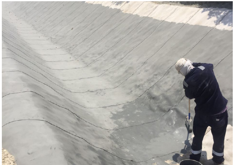
Painting completed installation
